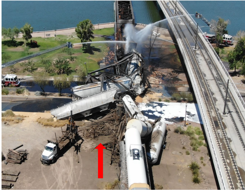
Figure 1. Aerial photo of the derailment site. Red arrow shows direction of train. Light rail operation to the east of UP's right-of-way.
