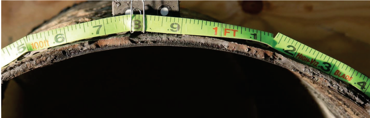
Figure 1: Photograph of fracture surface. Numbered scale divisions are inches.
