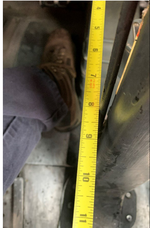
Figure 14. First Officer control column at rest location. The measurement from the footrest below the flight displays to the aft side of the control column (side facing FO seat). The measurement was 8.75 inches.
