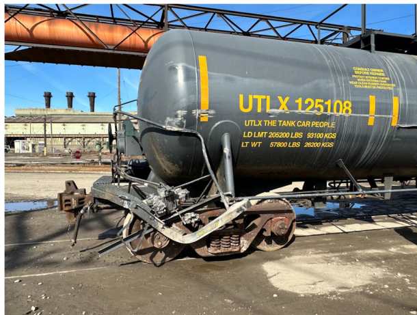
Figure 3 - Photo of damaged platform and steps on the railcar that was being ridden by the Conductor at the time of the accident (Photo courtesy of BLET)
