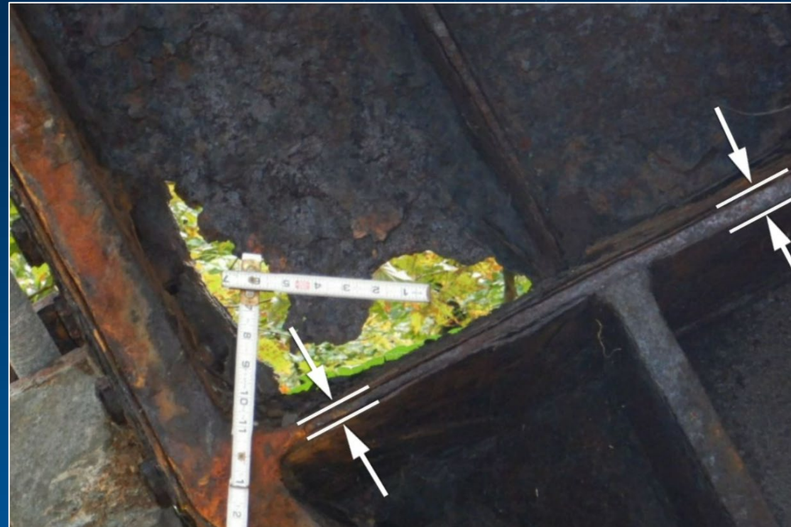
Source: 2021 inspection report
