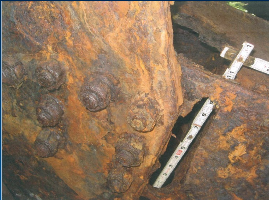
Source: 2005 inspection report
