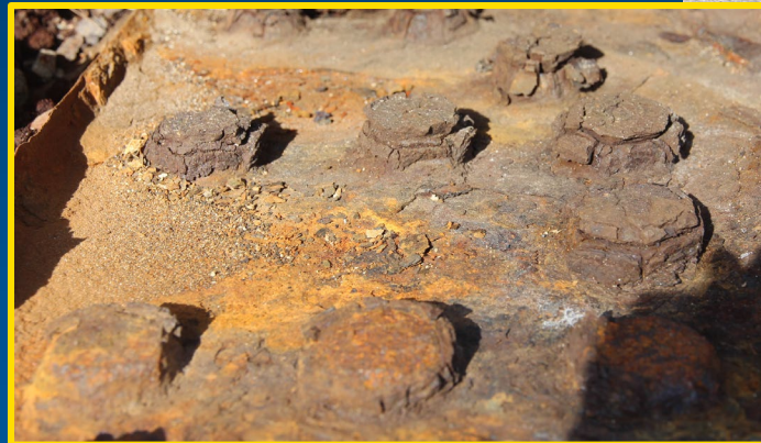
Rusted connecting bolts
