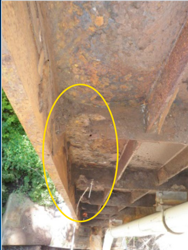
Source: 2013 inspection report
