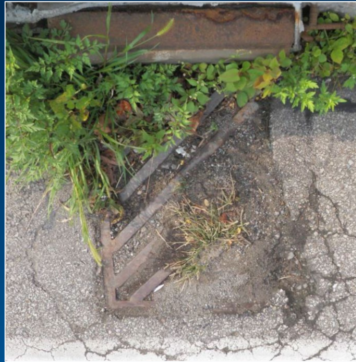
Source: 2017 inspection report
