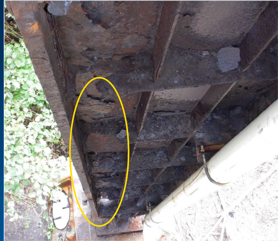
Source: 2021 inspection report
