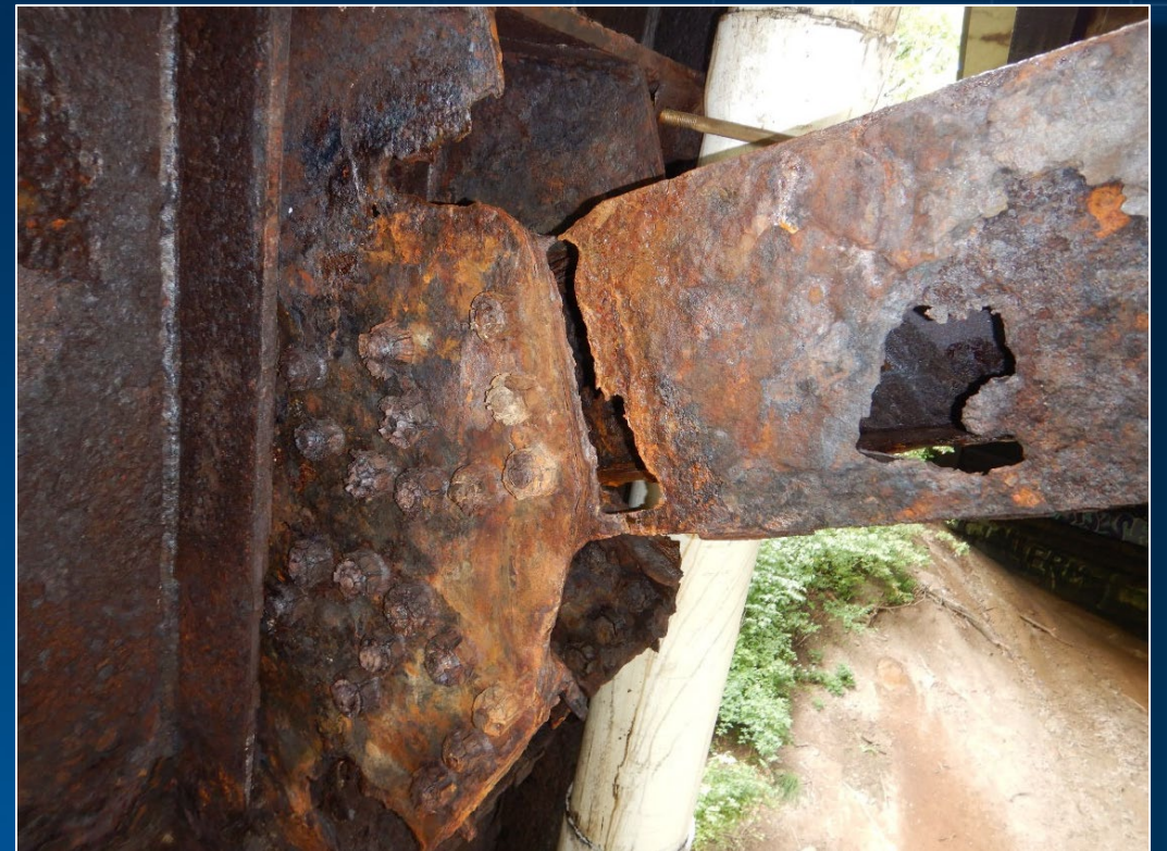
Source: 2021 inspection report
