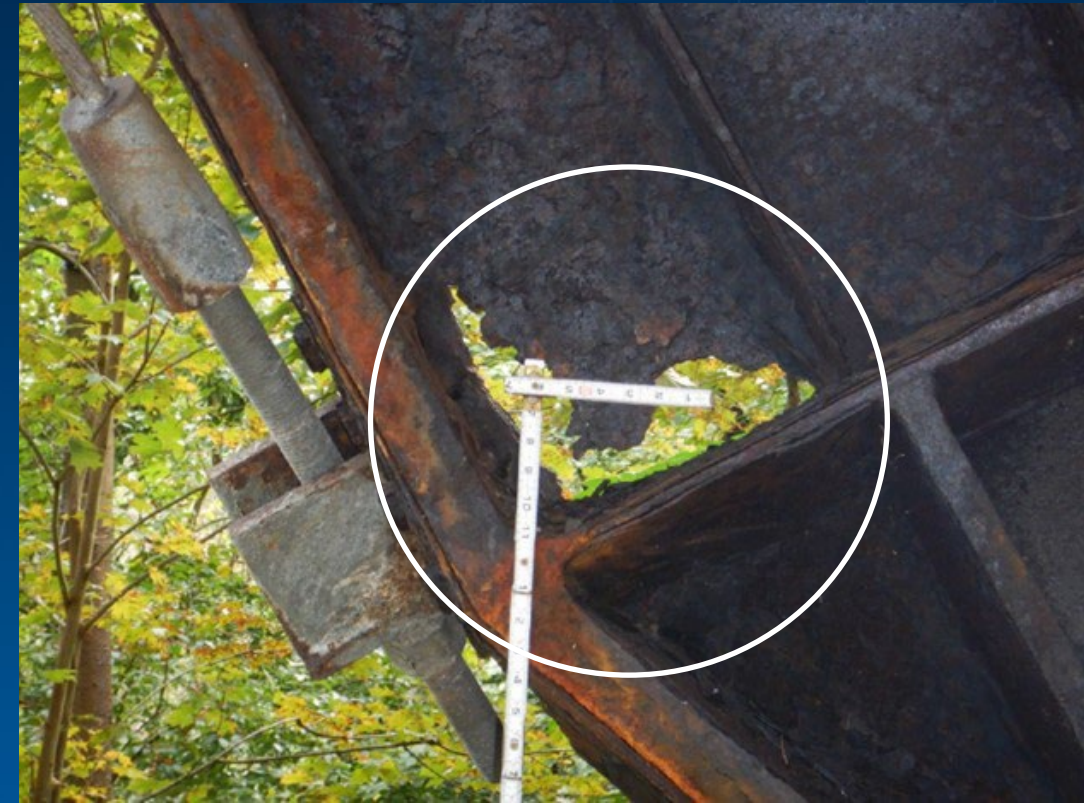
Source: 2021 inspection report
