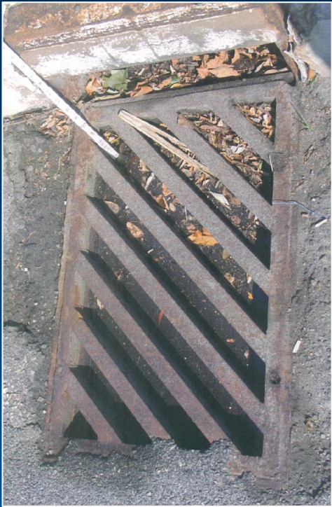
Source: 2005 inspection report
