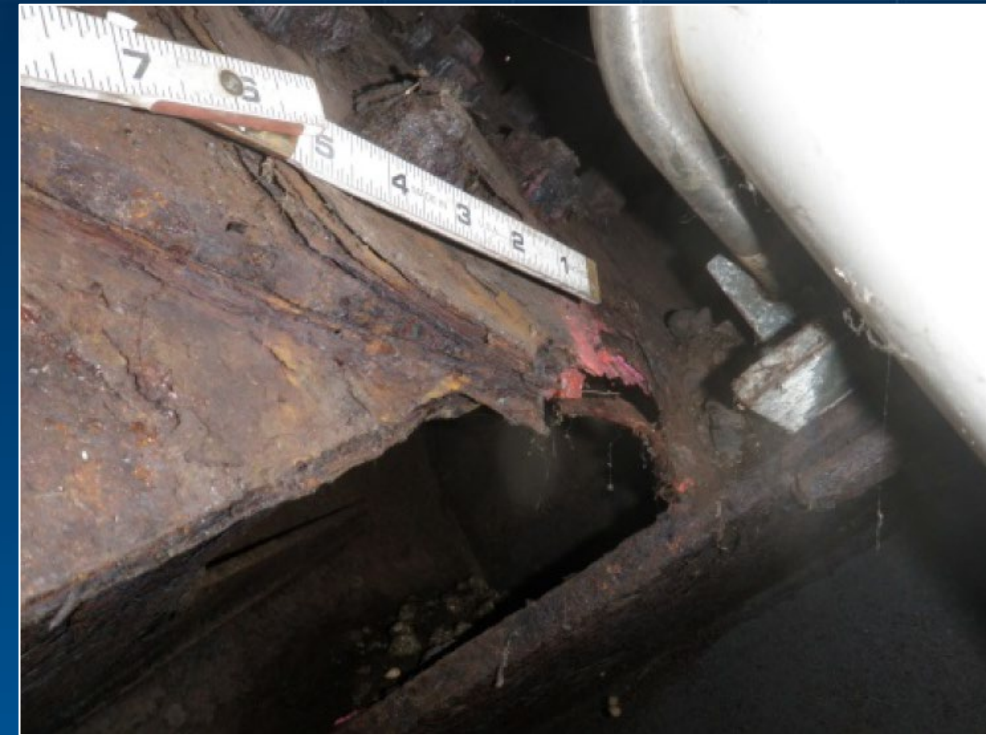
Source: 2015 inspection report
