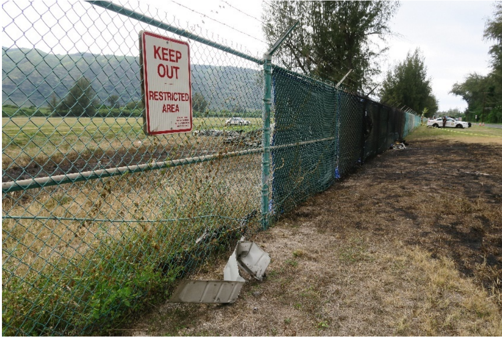
Figure 26. The unburned nose landing gear door was found on the street side of airport perimeter fence, visible beneath the KEEP OUT sign. A heat exchanger, portion of a main landing gear, and other debris is visible in background, farther away from the photographer. (Photo from: Textron)
