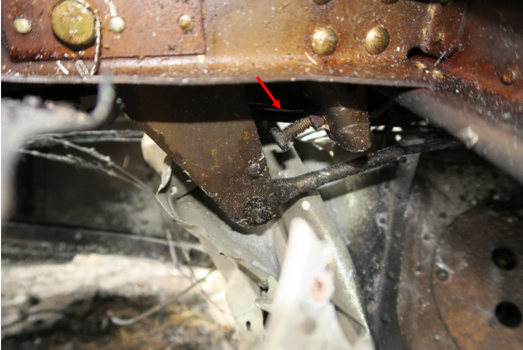
Figure 79. Left wing aileron control forward stop bolt found fully extended. (Photo from: Textron)
