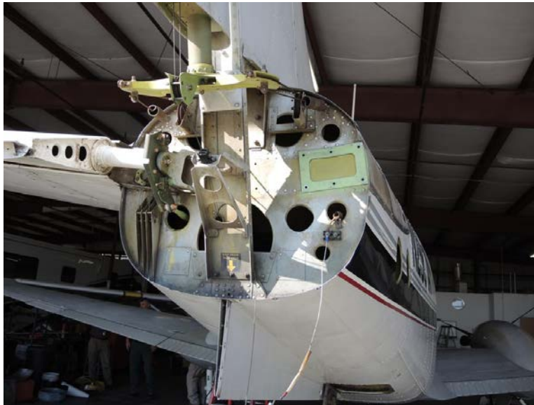
Figure 4. The rear tail bulkhead with the tail cone fairing removed. (Photo from: Textron Report ASI-16-CF, taken August 11, 2016)
