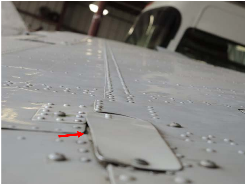
Figure 14. Compression buckle of thin aluminum fairing over rear wing attach fitting. (Photo from: Textron Report ASI-16-CF, taken August 11, 2016)
