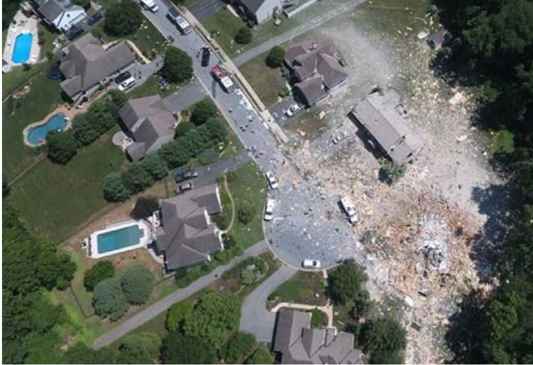
Figure 1. Debris field at cul-de-sac area where the explosion the occurred
