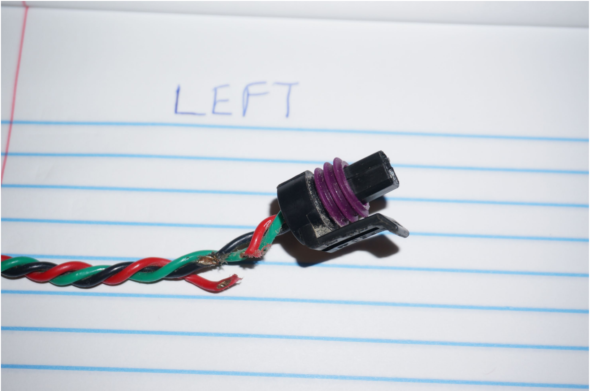
Photo 3 – Close Up of Left Wiring Harness
