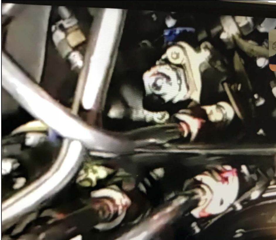
Photo 2: View of the fuel and air lines
