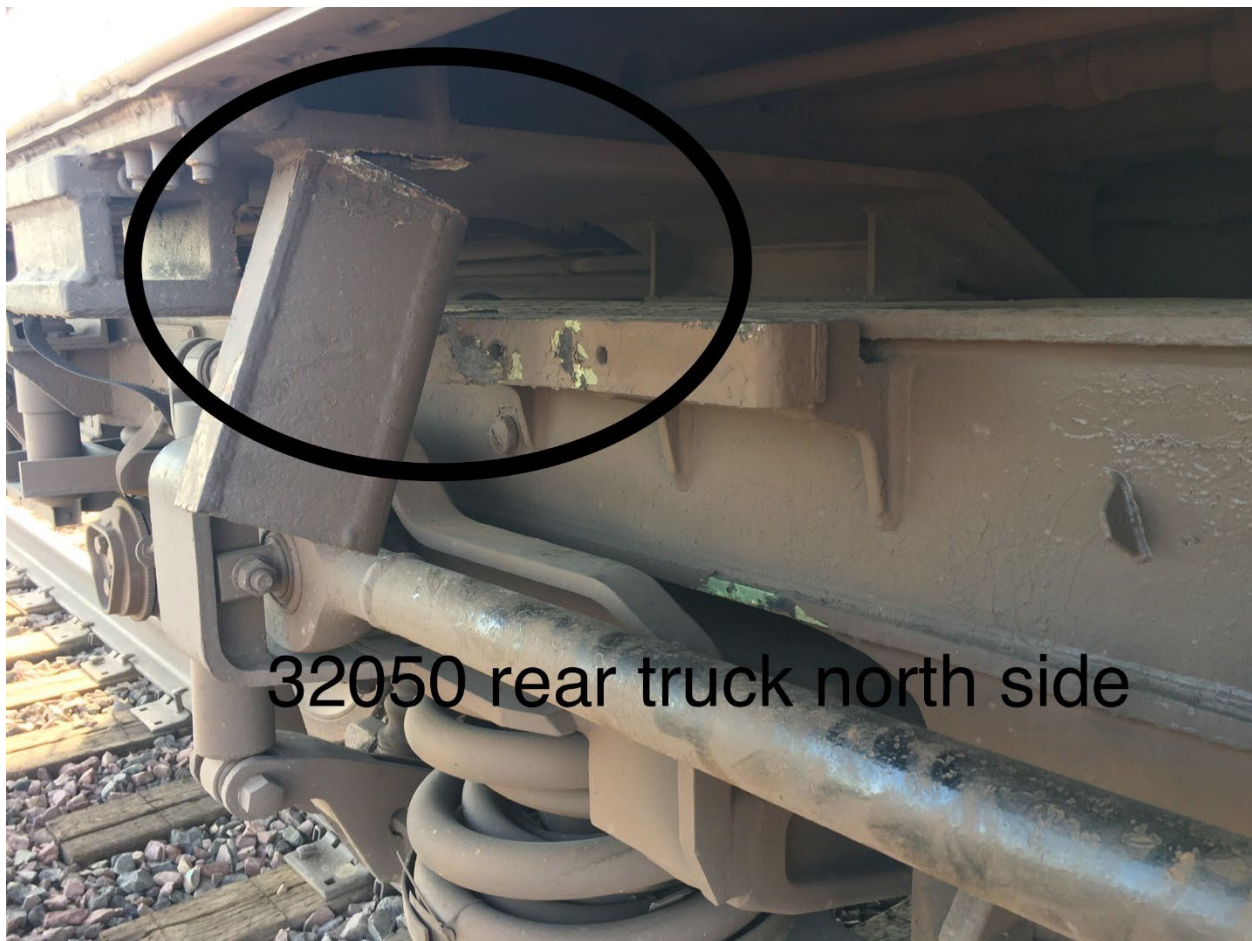
Figure 6. Photograph of the 32050 north side truck, showing bump stop damage. This photograph was taken by and annotated by Volpe staff while on scene. The north side corresponds to the right side of the train and the right side of the car. (Low rail)
