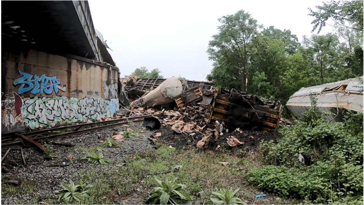
Figure 4. Derailed cars on the Norfolk Southern tracks.
