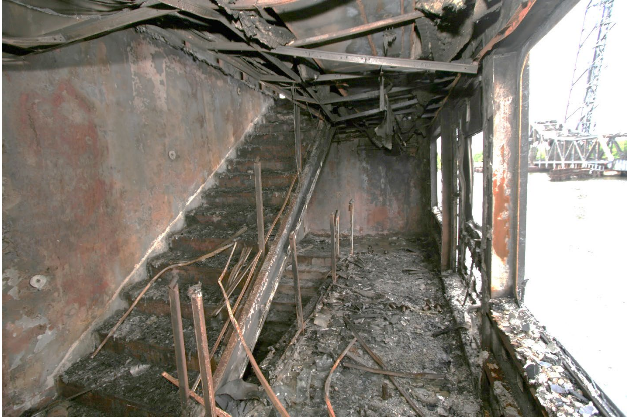
Figure 13. Stairwell from second deck to the third deck.
