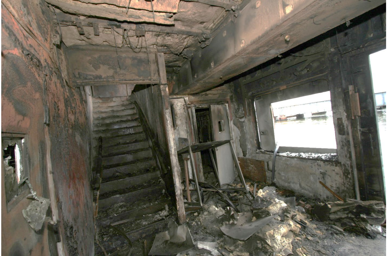
Figure 12. Stairwell from main deck to second deck including passenger boarding area.
