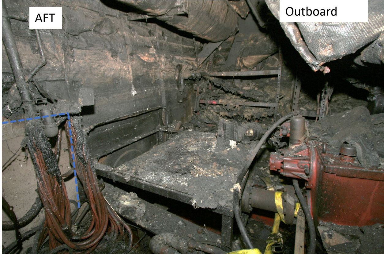
Figure 22. Bulkheads aft and outboard of port main engine.
