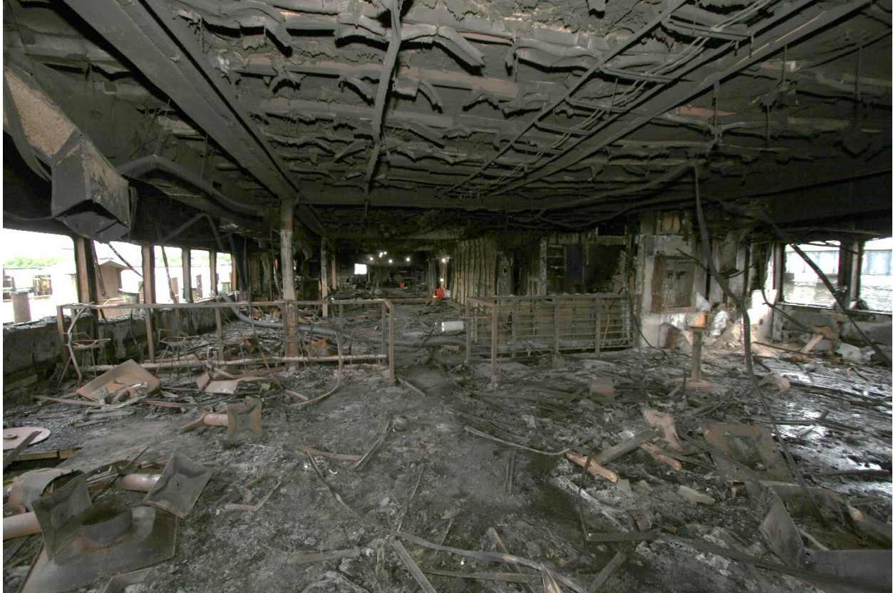
Figure 5. Main deck interior looking aft.
