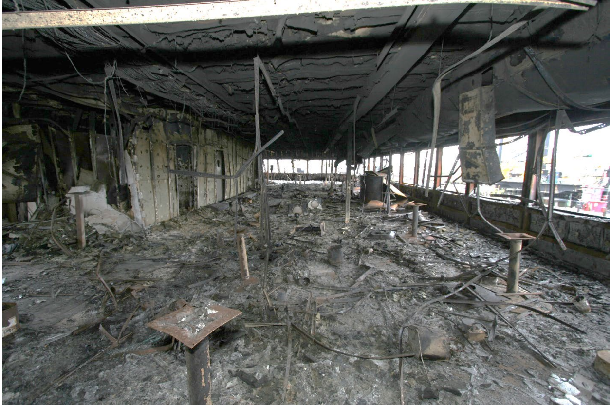
Figure 7. Second deck interior looking forward.
