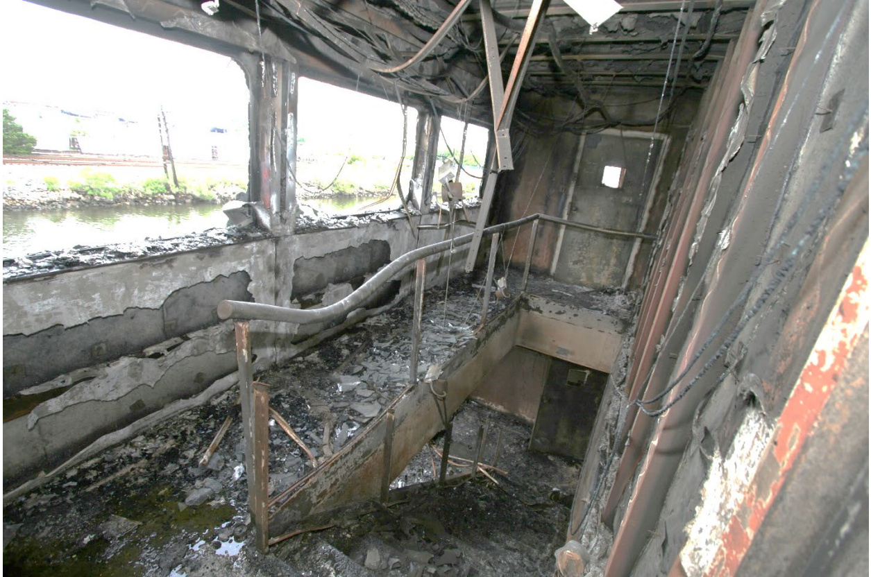
Figure 14. Stairwell on the third deck looking forward towards wheelhouse door.
