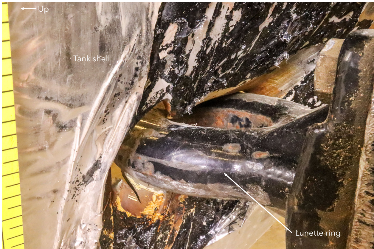
Figure 13. Closer view of the perforation in the exterior side of the front head shell piece with the trail hitch lunette ring placed close to the perforation.
