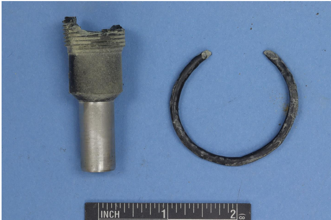
Figure 3. The cutter and O-ring, recovered from the excavation site for the active and retired service tees that provided gas service to 17 S. 2 nd Ave (Palmer building #2).
