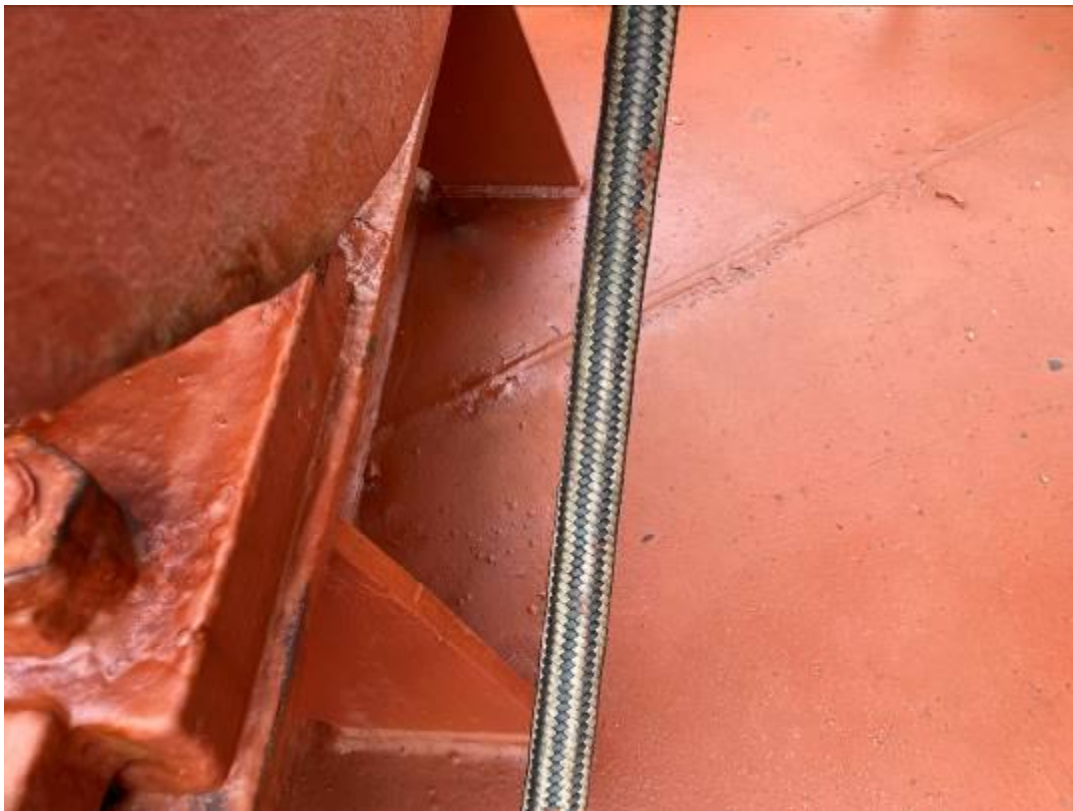
38. Close view of Mooring winch HMPE-Polyethylene rope located at starboard side forward mooring station.
