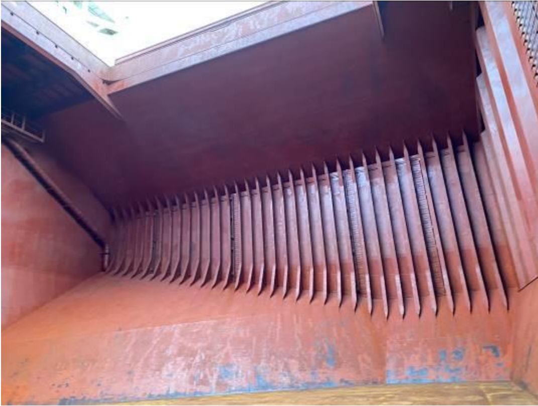
103. Hold #7 - Port side bulkhead.
