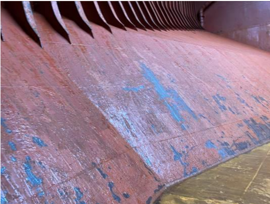
104. Hold #7 - Starboard side lower hopper slope.
