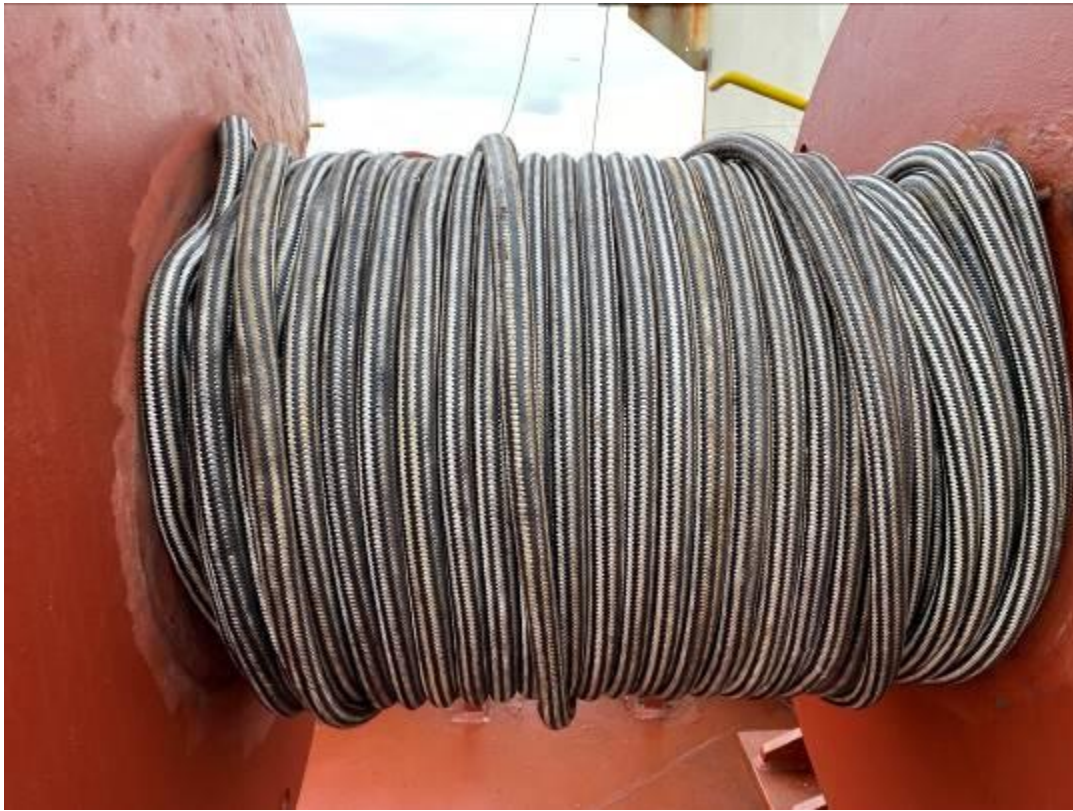
37. Close view of Mooring winch HMPE-Polyethylene rope located at starboard side forward mooring station.
