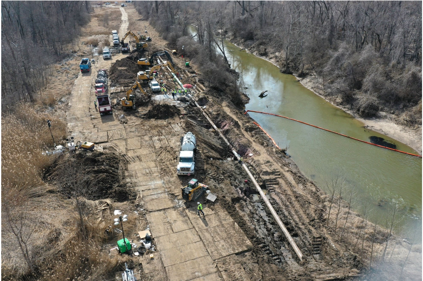
Figure 14. Source area remediation activities and pipeline reconstruction. March 14, 2022, 3:43 p.m.
