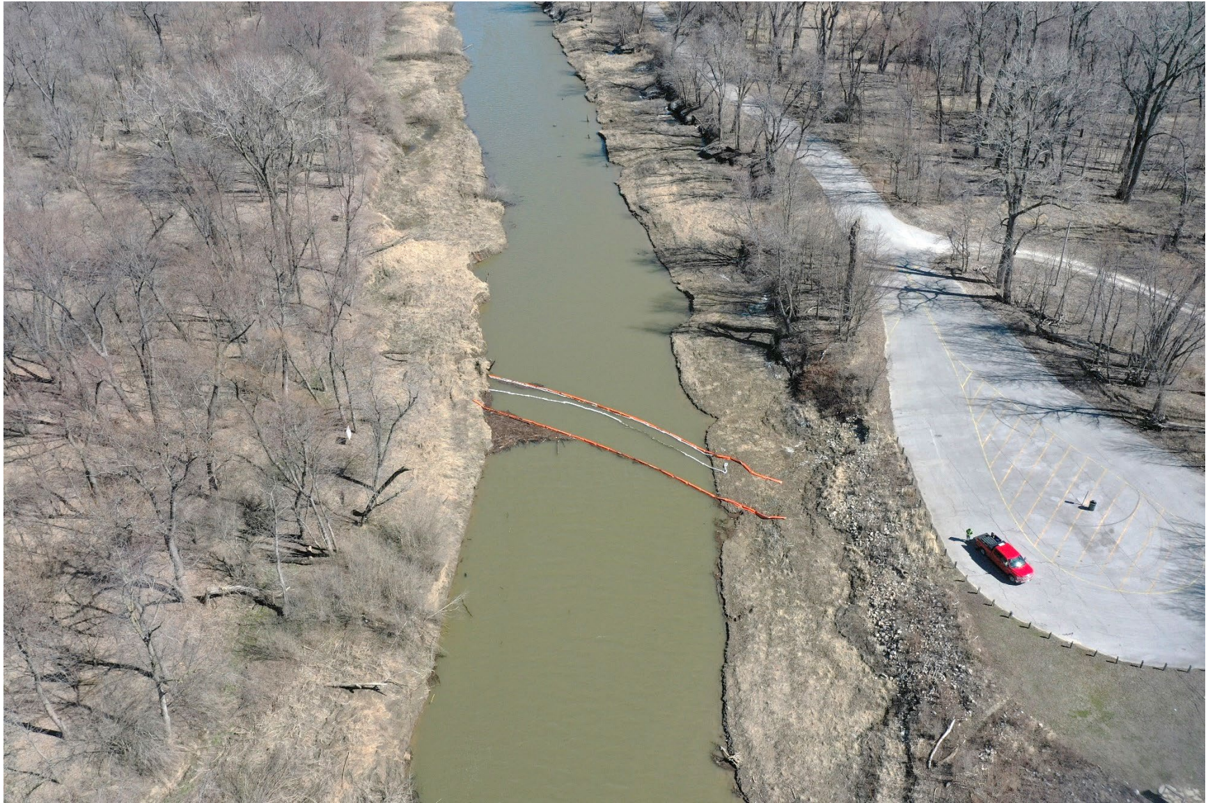
Figure 11. Division 4 oil boom on Cahokia Creek, East of Mississippi River. March 12, 2022, 1:09 p.m.
