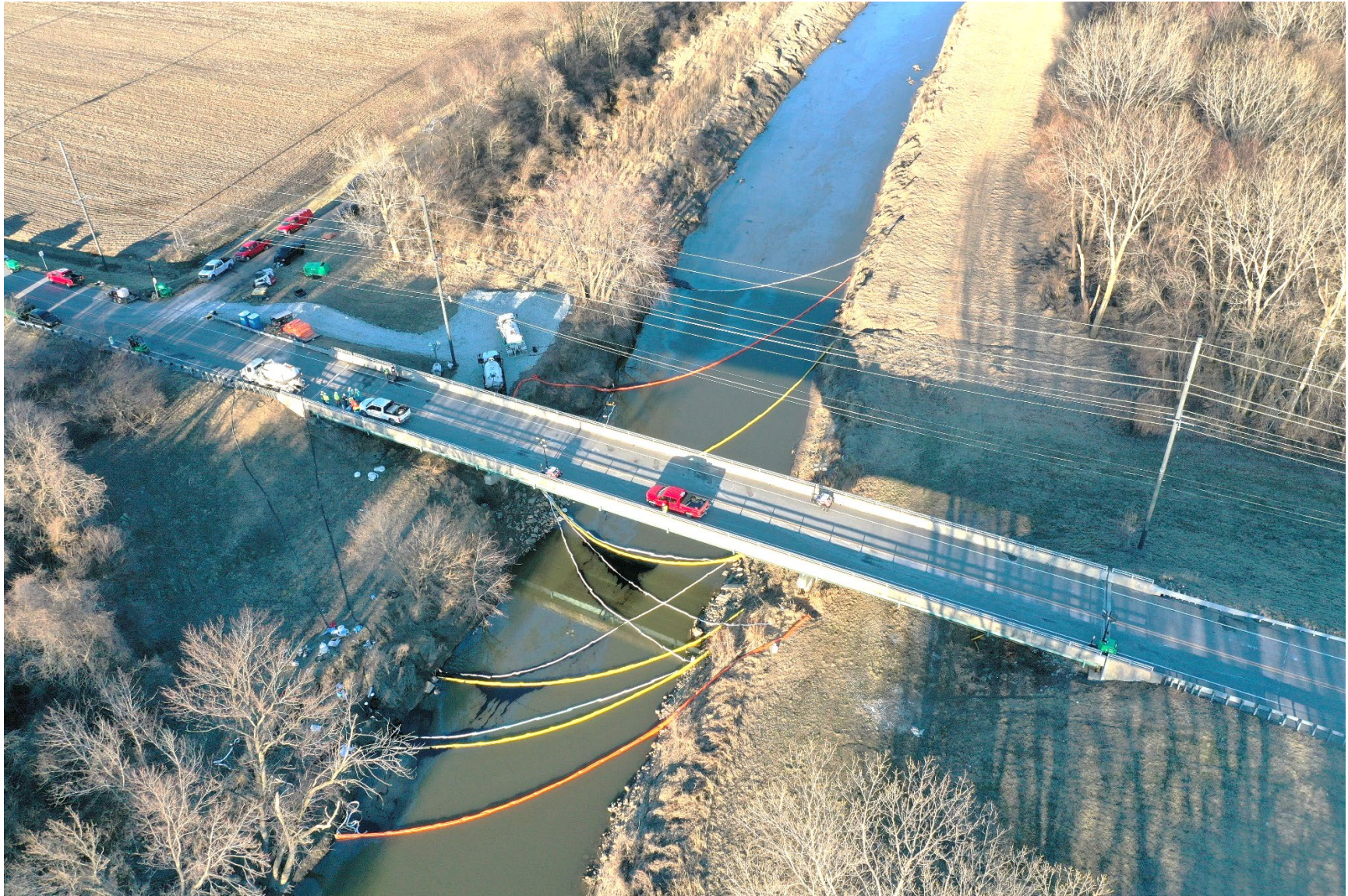
Figure 6. Division 2, Cahokia Creek at Wanda Road bridge. March 12, 2022, 5:05 p.m.
