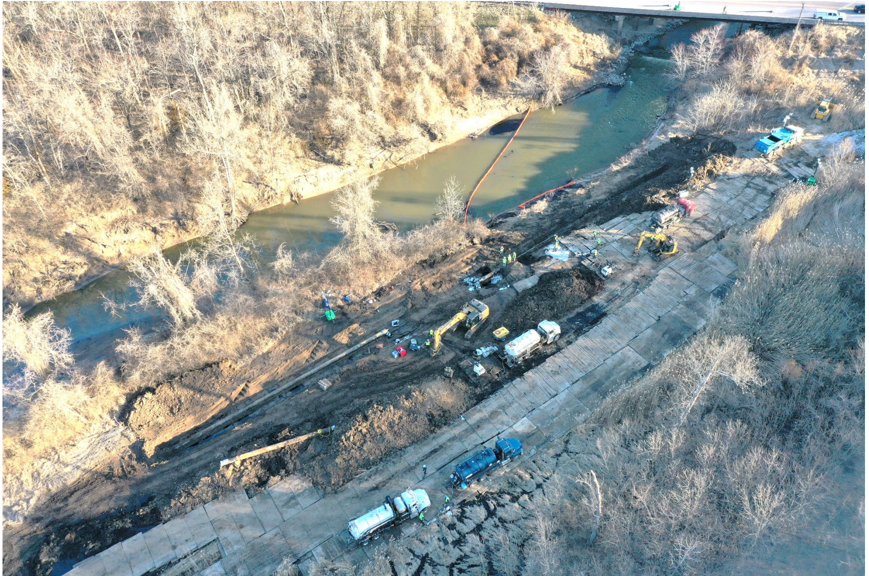
Figure 3. Division 1, source area operations. March 13, 2022, 08:20 a.m.
