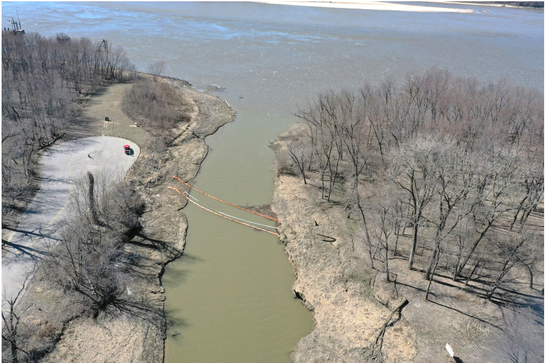
Figure 12. Division 4, oil boom site on Cahokia Creek east of the Mississippi River. March 12, 2022, 1:10 p.m.
