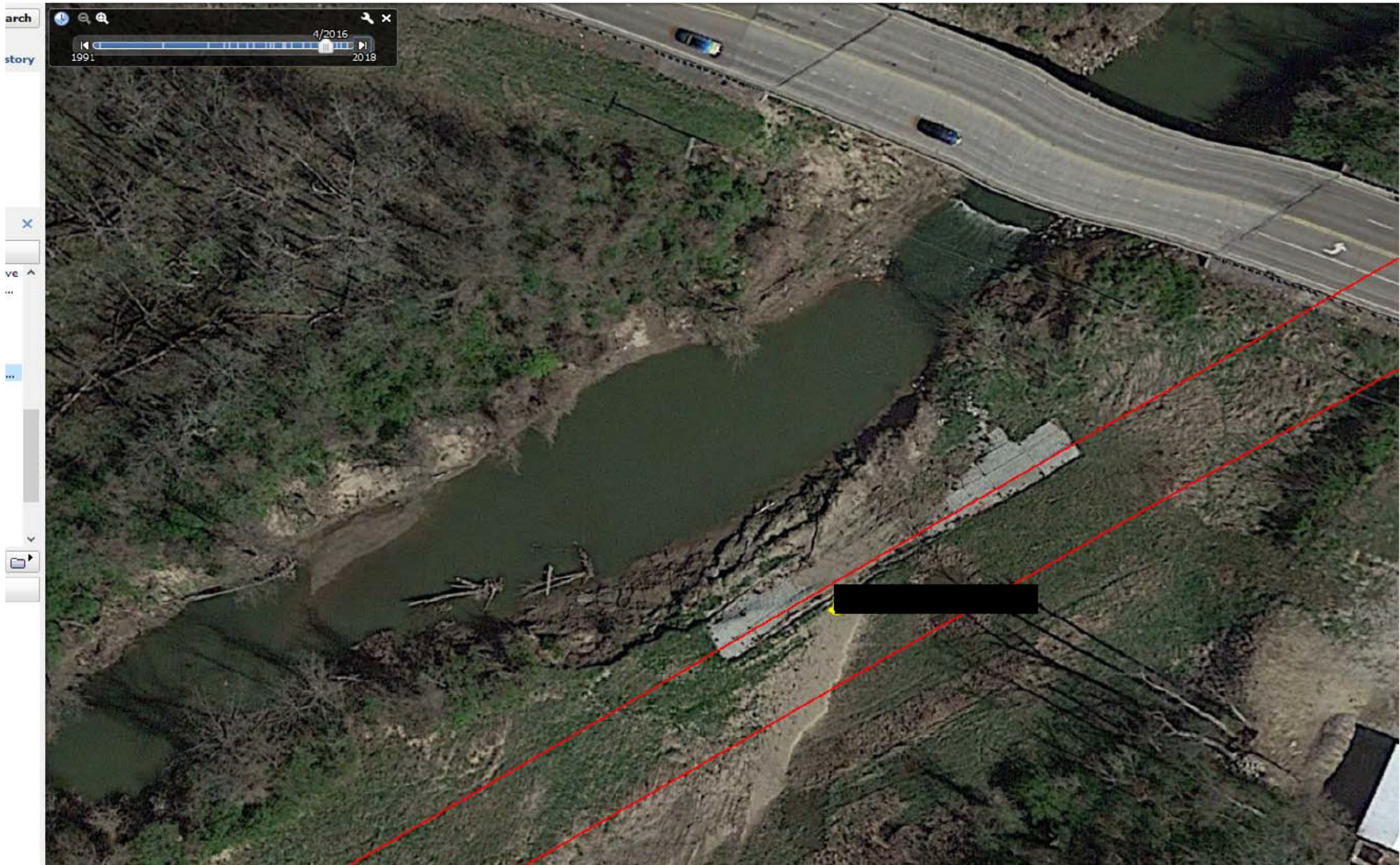
Mats were installed at this waterway encroachment in 2015 as a P&MM.
