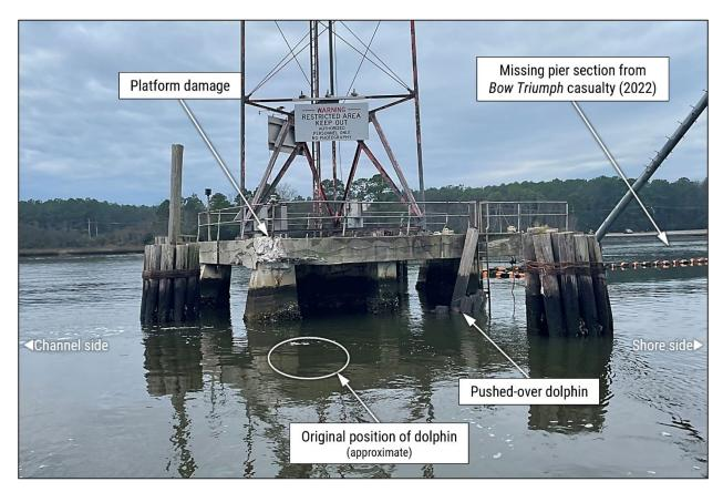
**Figure 6.** Naval Weapons Station Pier B, showing damage to the platform and protective dolphin.
