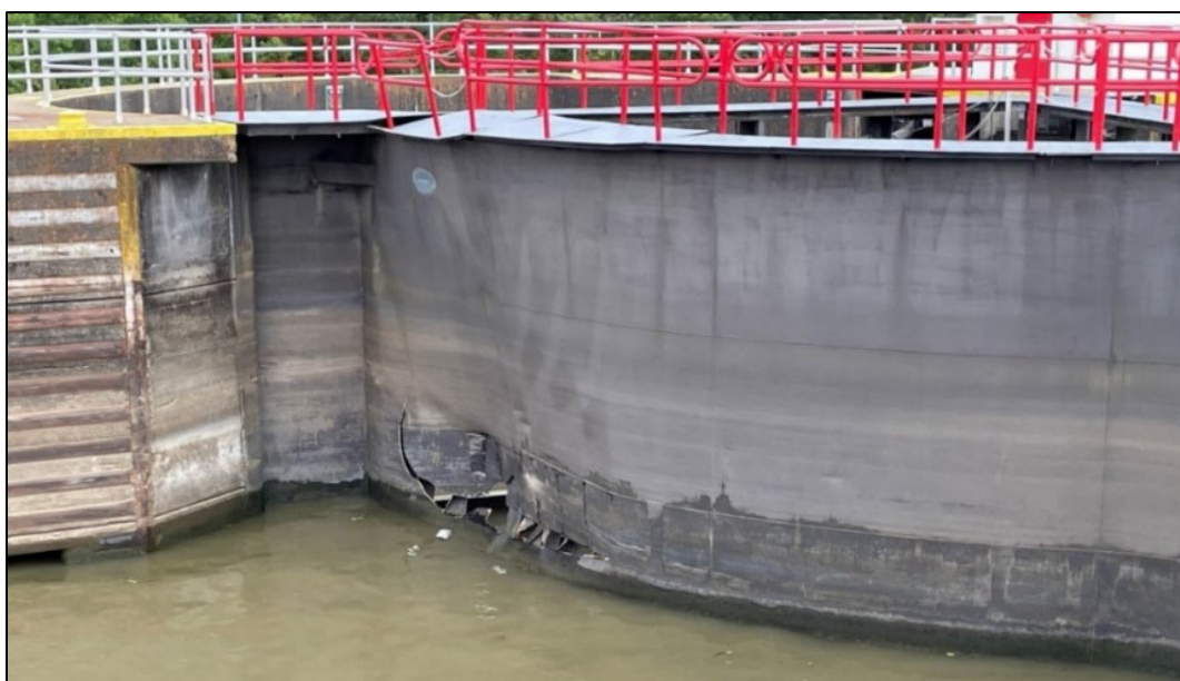
Figure 8. Damage to Gate D as viewed from the north wall of the lock chamber.
