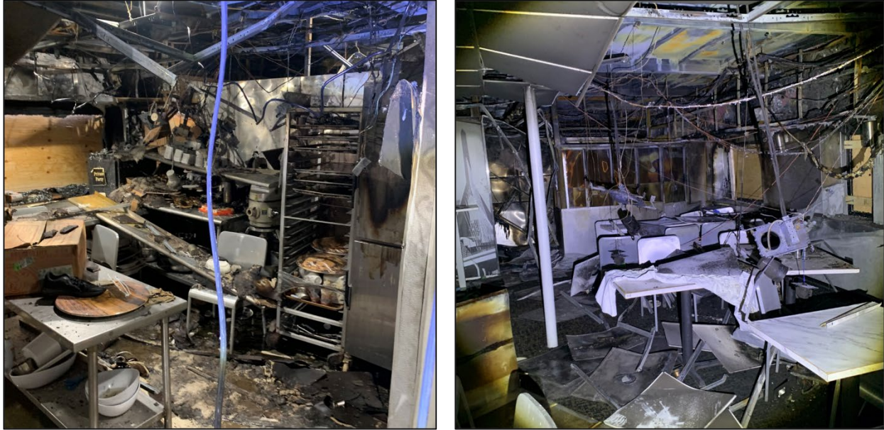
Figure 11. Left to right: Port side of the Spirit of Boston cold prep room, aft of the deck 1 wait station, after the fire, looking forward. Port aft corner of the passenger area on deck 1, forward of the wait station, after the fire.
