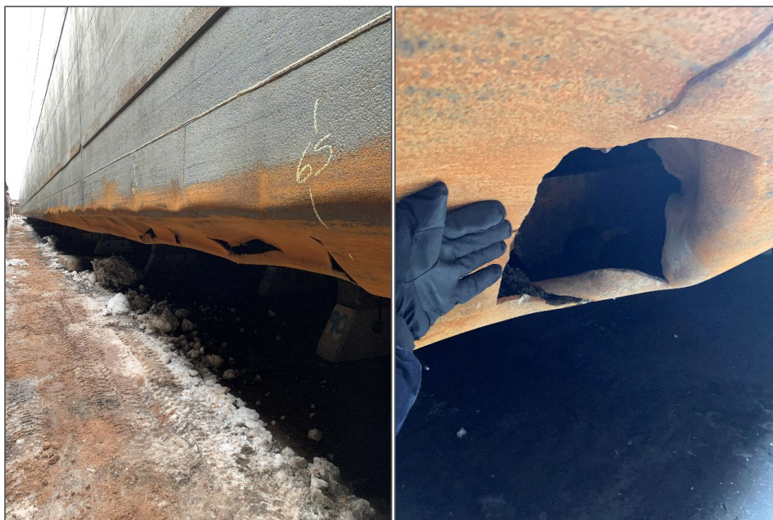
Figure 5. Damage to the port water ballast tanks. (Source: Coast Guard)
