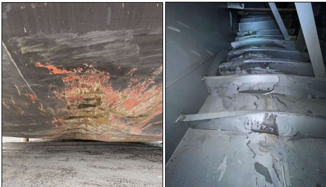
Figure 5. Left to right: Damage to the bottom of the Jungjuk's hull looking aft along the centerline and damage to the barge's internal structure and framing. (Source: Coast Guard)
