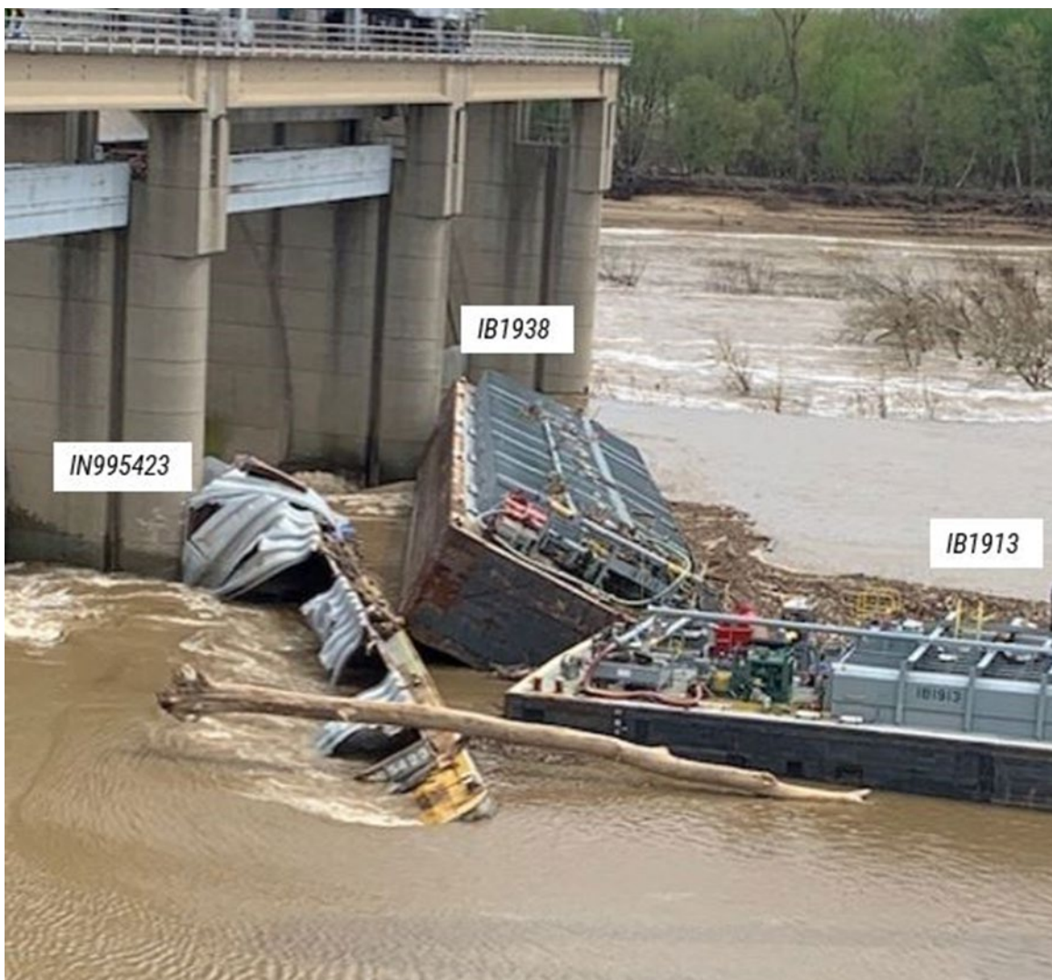
Figure 6. Barges IN995423 and IB1938 against the lower dam gates. IB1913 is receiving methanol from IB1938 through a cargo transfer hose. (Background source: Coast Guard)
