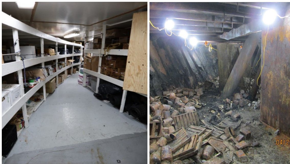
Figure 10. Left to right: The dry stores room, looking forward, before and after the fire. (Sources: Trident Seafoods, Coast Guard)
