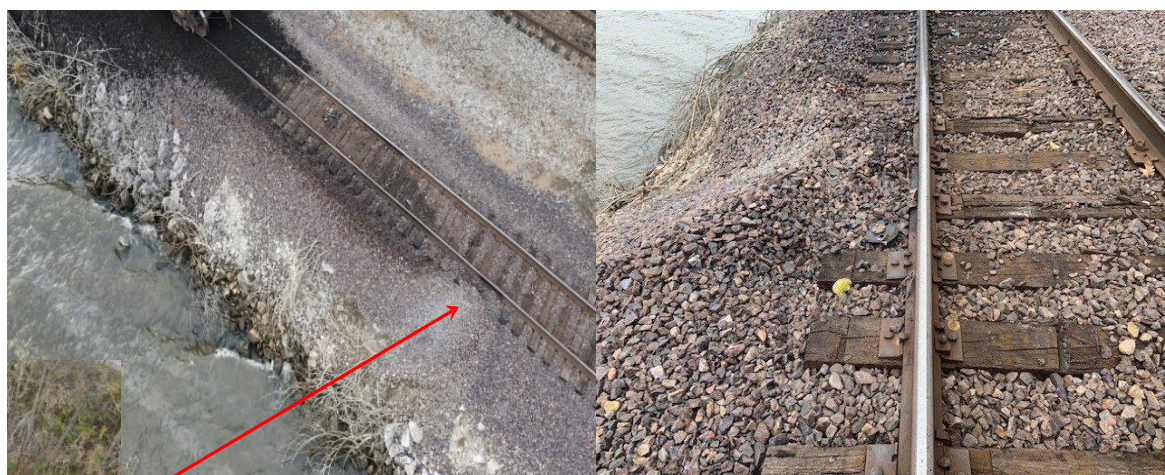
Figure 8. Aerial drone photo of the casualty site with a red arrow pointing to the indentation remaining in the ground where the forwardmost barge STC 3020 was located ( left ). Close-up of the indentation from the barge in the shoreline next to the railroad track ( right ). (Sources: BNSF [ left ], Coast Guard [ right ])
