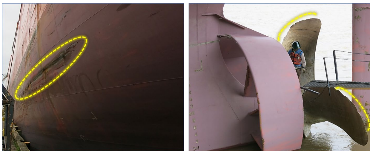
Figure 6. Postcasualty damage to the Bow Tribute 's portside aft hull ( left ) and propeller ( right ), as indicated by yellow dashed lines.
