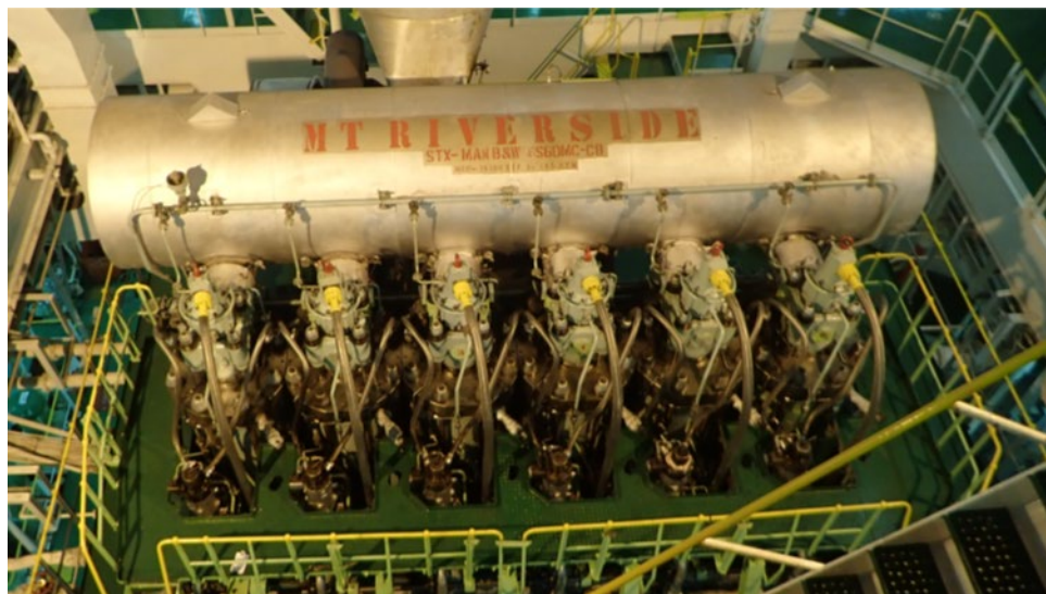
Figure 8. The top of the Riverside main engine. (Source: Coast Guard)
