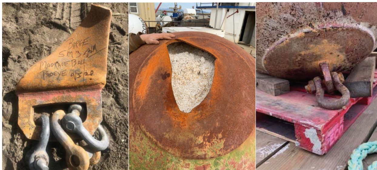
Figure 7. SM-3 mooring buoy: failed padeye (with three shackles) that separated from buoy (left), damaged top with padeye missing (center), and undamaged bottom padeye (right). (Source: Alaska Marine Surveyors and Northline Seafoods)
