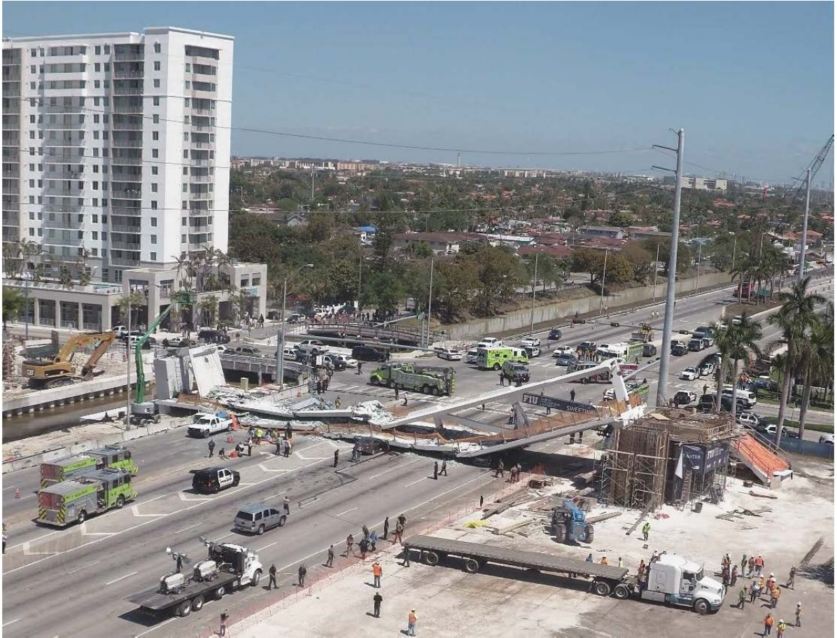
Figure 8. Aerial photo of collapsed Main Span and rescue efforts. 29
