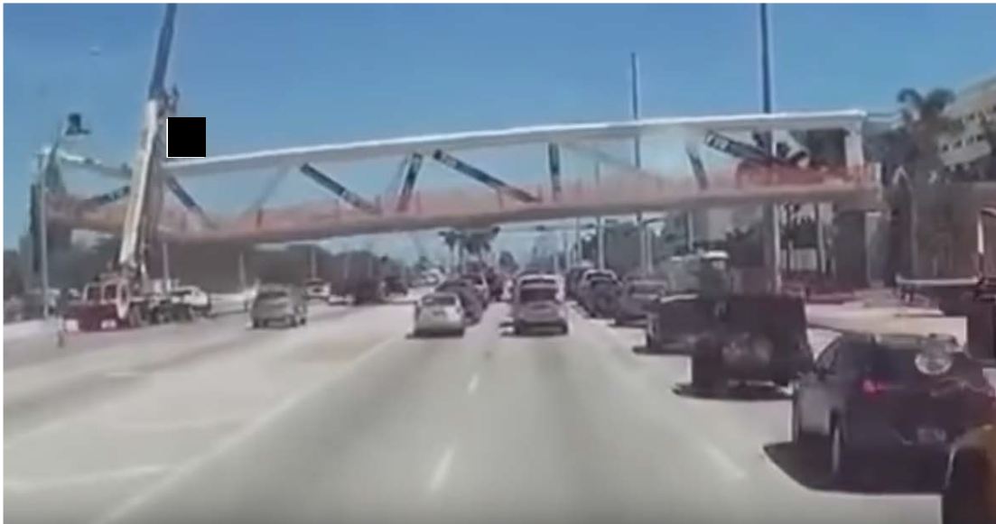
Figure 7. Frame from dashboard video of Bridge collapse. 28
