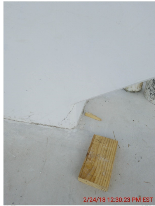
Figure 36. Cracks documented on February 24, 2018, before complete removal of shoring. 121
