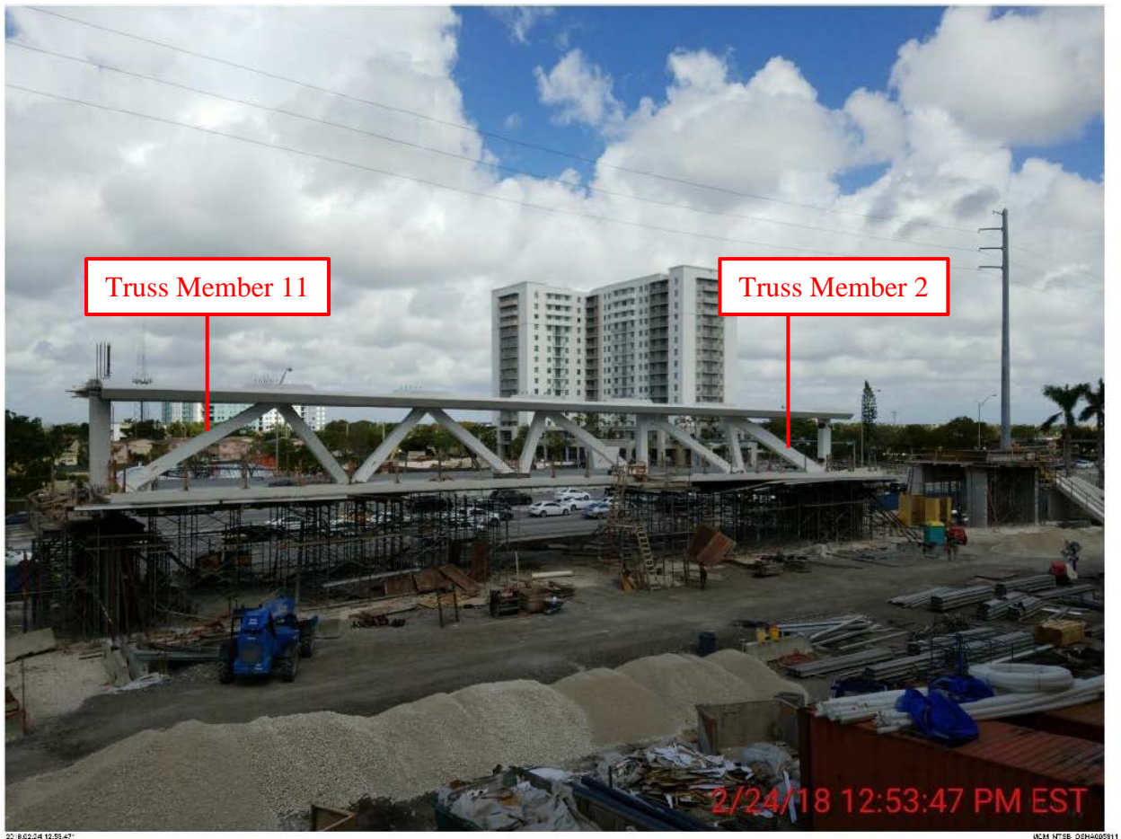
Figure 34. Photograph of Main Span taken on February 24, 2018. 113
