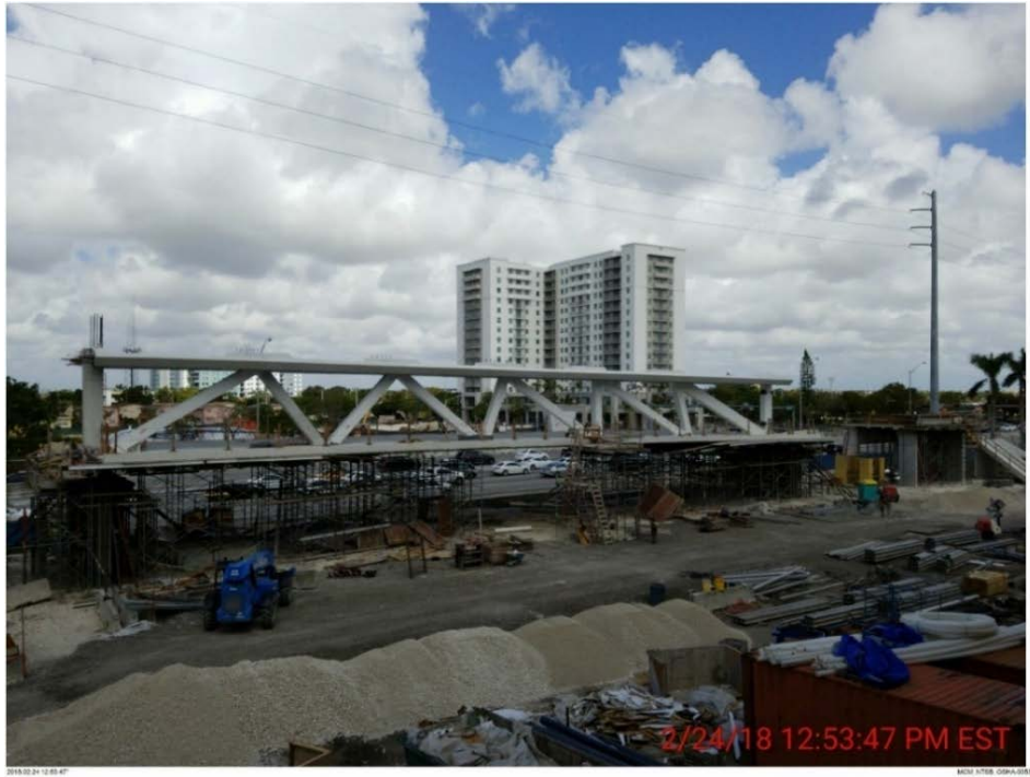
Figure 28. February 24, 2018: Formwork and shoring removal. 87
