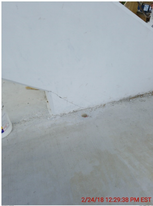
Figure 36. Cracks documented on February 24, 2018, before complete removal of shoring. 121
