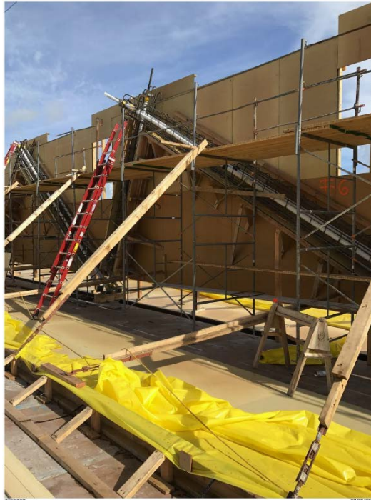
Figure 18. July 7, 2017: Deck and Truss forms. 77
