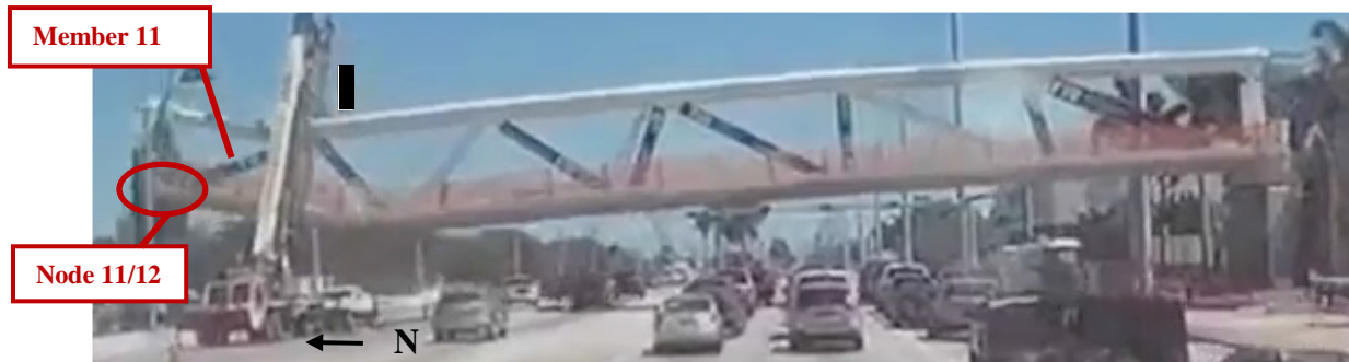
Figure 1. Frame from dashboard video of Main Span during collapse, showing that the failure originated near the north end of the Main Span. 1
