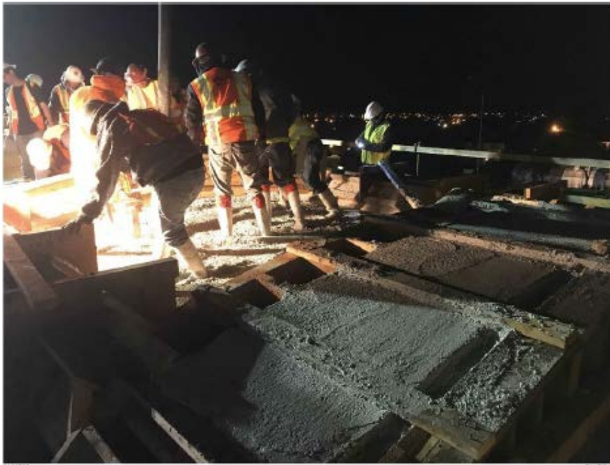
Figure 25. December 14, 2017: Canopy concrete placement. 84
