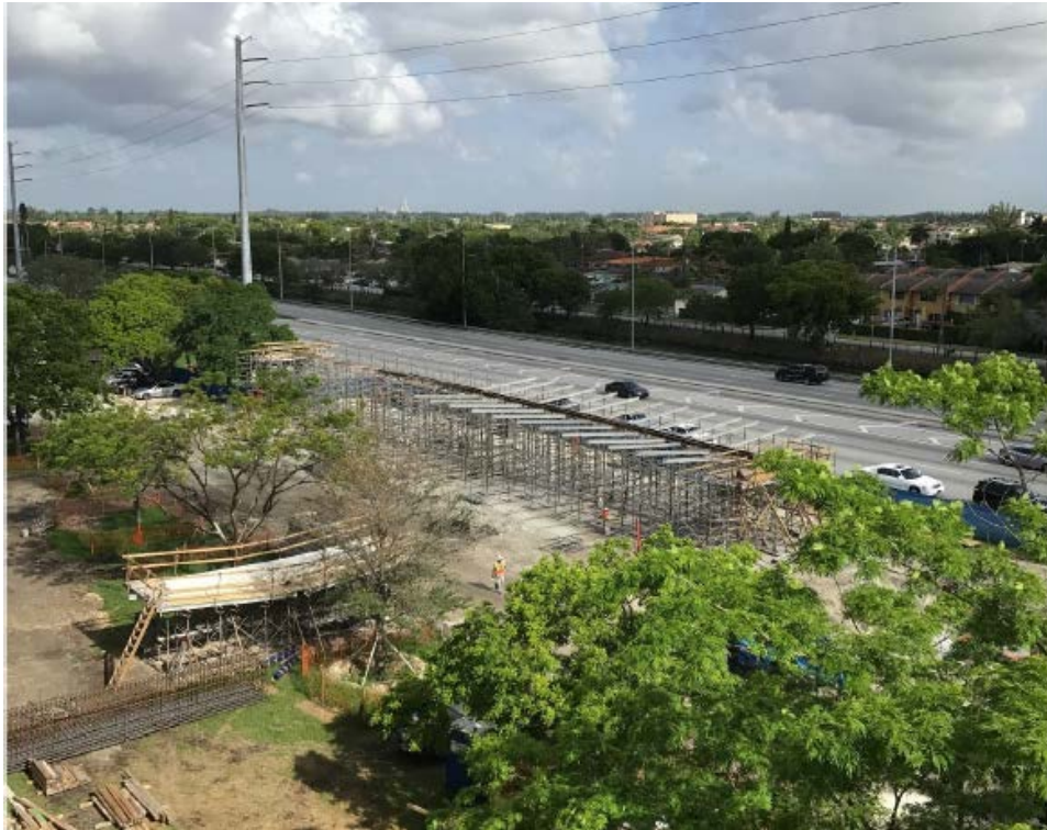
Figure 17. May 30, 2017: Erection of shoring and forms for Main Span. 76
