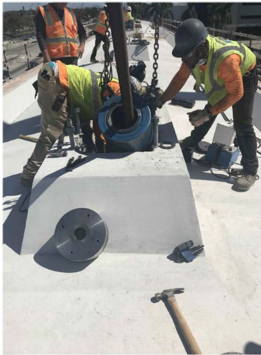
Figure 27. February 17, 2018: Truss post-tensioning. 86
