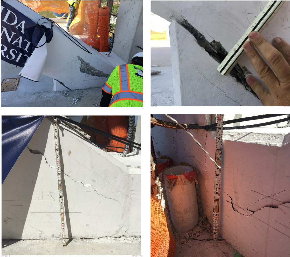
Figure 57. Northward displacement of Node 11/12 relative to Deck. 200
