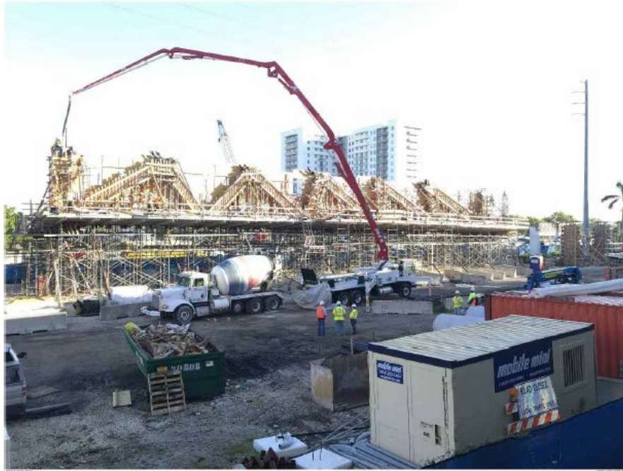
Figure 22. November 6: 2017: Truss concrete placement. 81
