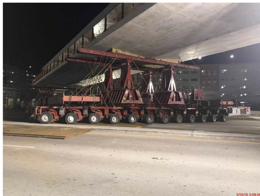
Figure 38. SPMT transport of Superstructure Main Span on March 10, 2018. 126
