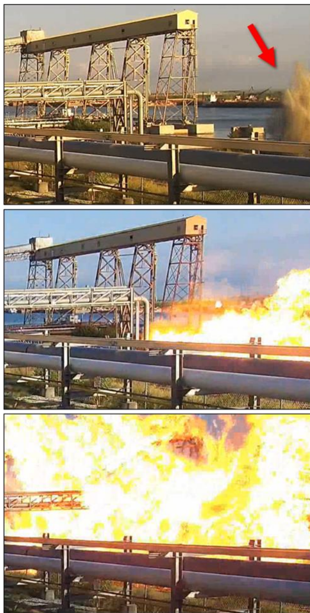
Figure 10. Screen captures from security camera footage showing, from top to bottom, the water and gas eruption before the explosion (as noted by red arrow), the initial explosion, and the ensuing fireball. The Waymon Boyd is outside of the frame of the camera. (Source: EPIC Crude Terminal Company)
