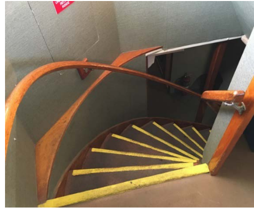
Figure 28. Staircase from the main deck galley/salon leading down to the bunkroom on the Conception . (Source: NTSB eyewitness submission)
