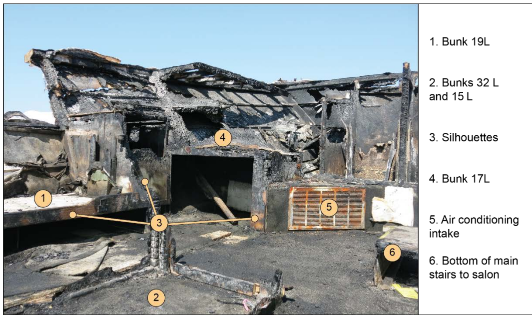
Figure 22. Postaccident photo of the bunkroom looking from the starboard aisle forward and to port.
