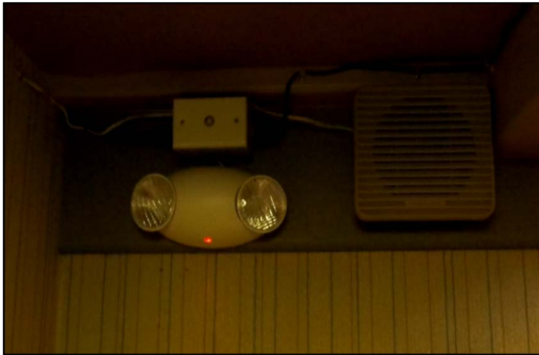
Figure 14. Bunkroom emergency lighting on board the similar vessel Vision . The lighting was of the same make and in a similar location as was on board the Conception . Also note the public address system speaker to the right of the lights.
