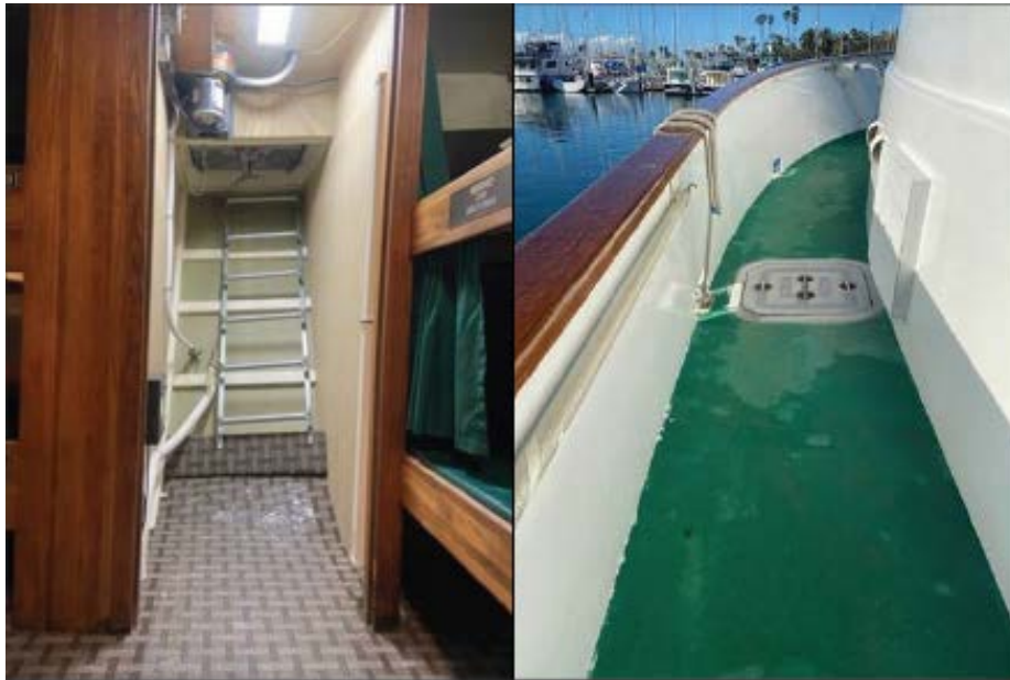
Figure 32. Modifications made to the Vision after the accident on the Conception . Left: Ladders at the forward end on each side of the bunkroom lead directly to the weather deck. Right: Flush-mounted watertight hatches were installed in the deck, outboard of the galley. (Source: Truth Aquatics)
