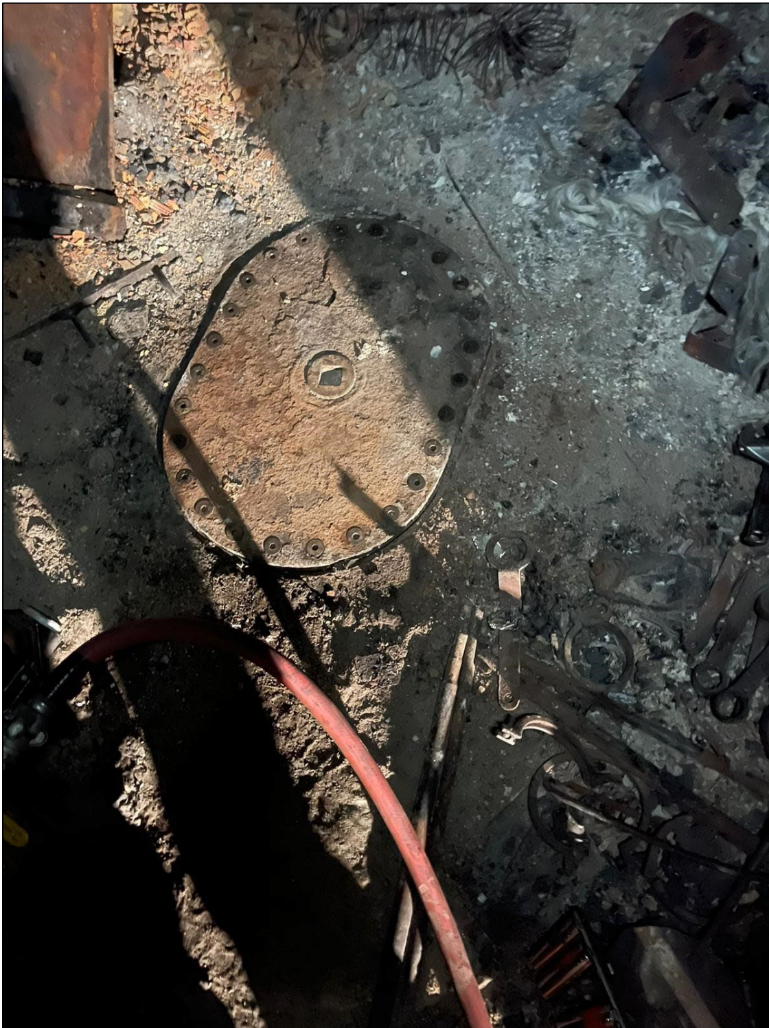
Figure 3 - Hatch covers reinstalled after clearing tanks 1 port and 1 starboard
