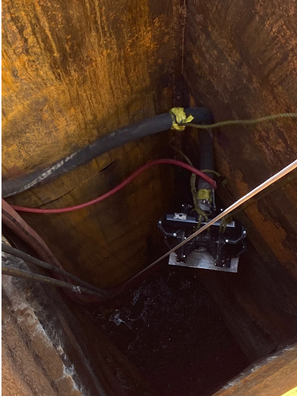
Figure 3 - Dewatering pump suspended in the hold of the vessel
