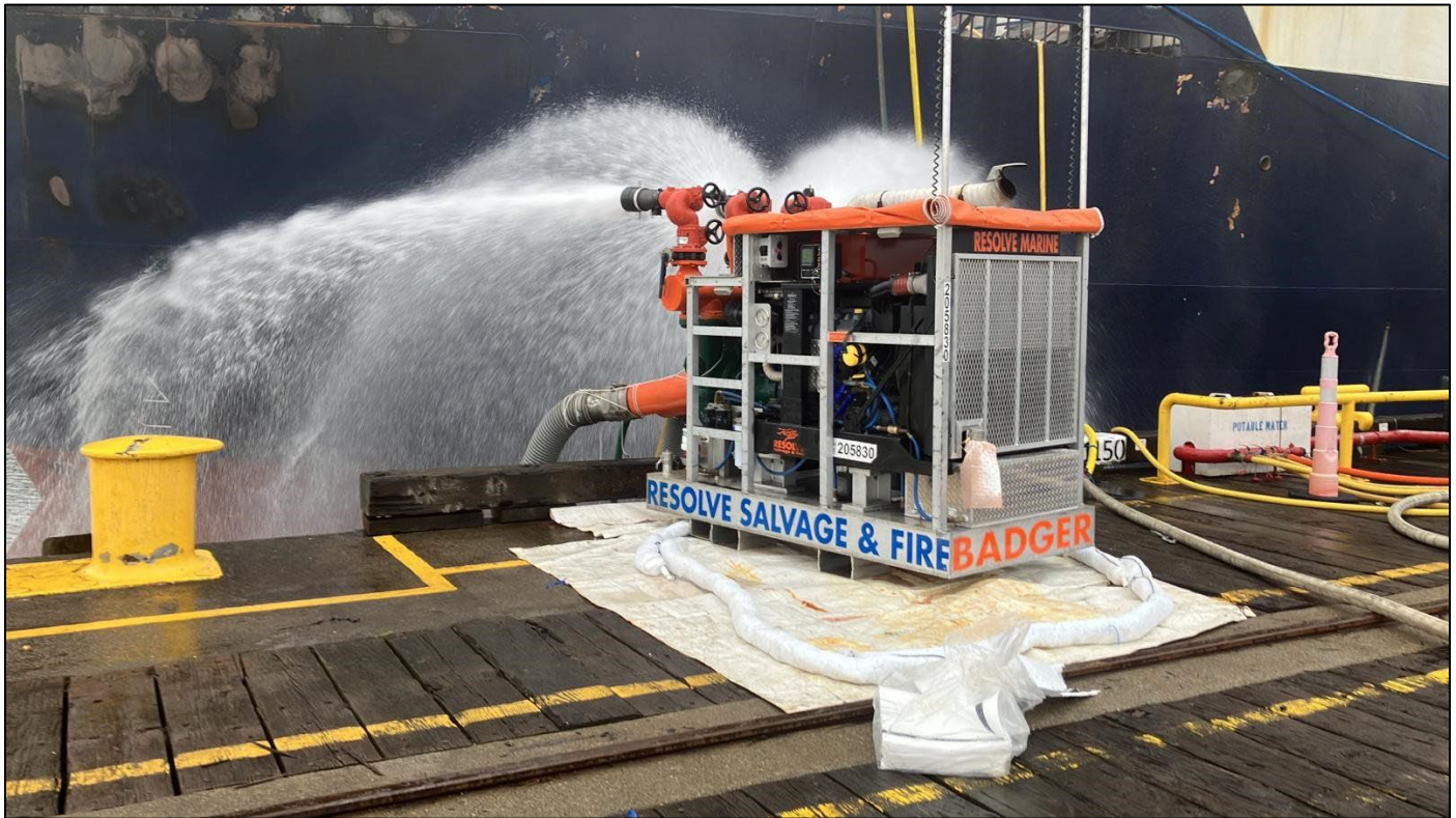
Figure 3 Resolve Fire Pump fired up.
