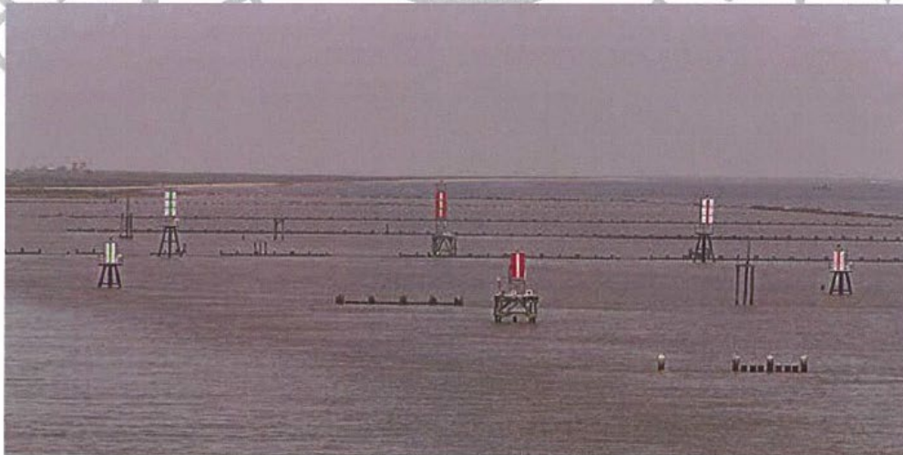
Southwest Pass Leading Lights B (8.55)
