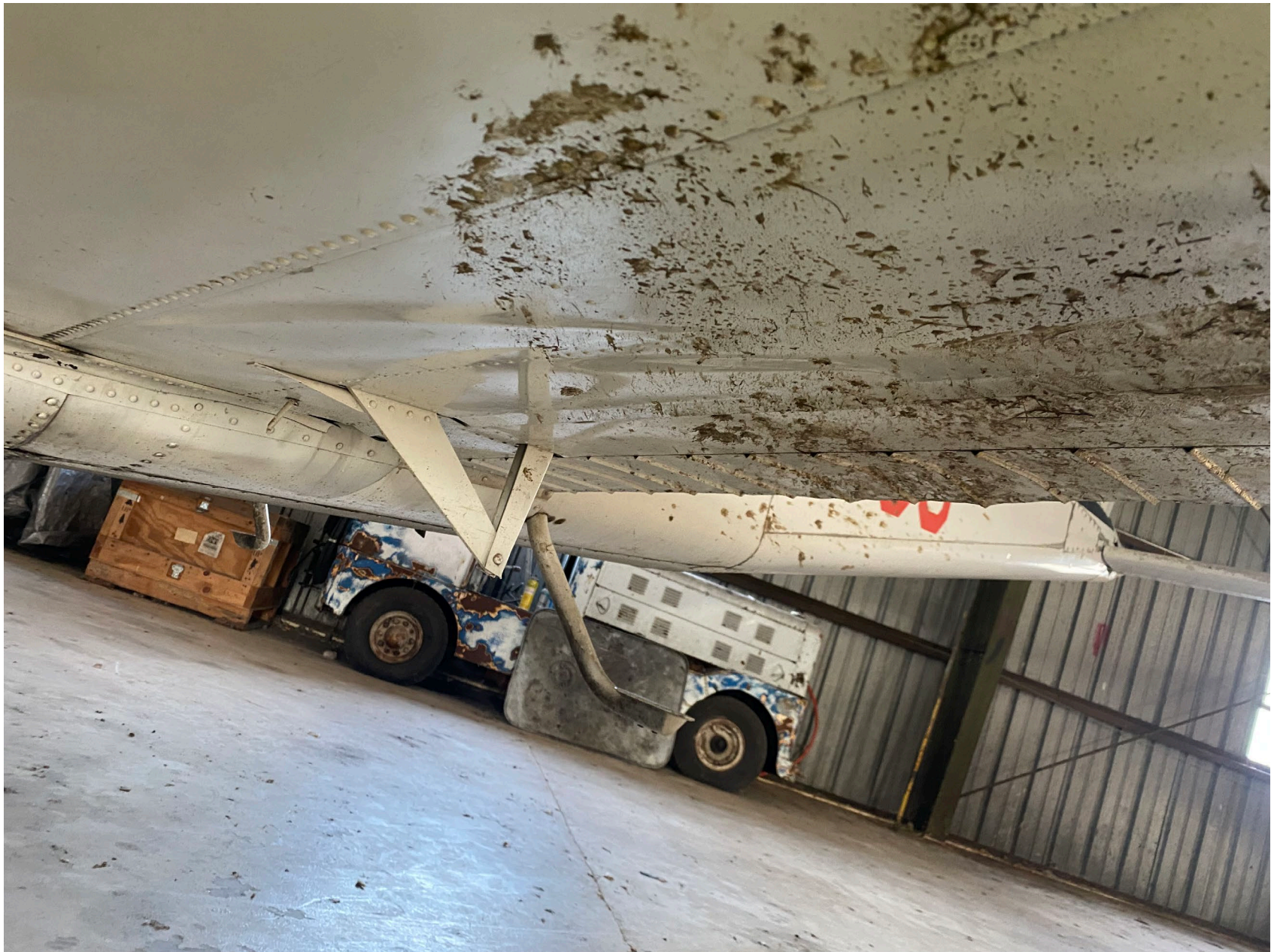
Photo 3 - FAA Digital Photograph. View Depicting the Wrinkles in the Lower Skin of the Left Wing.
