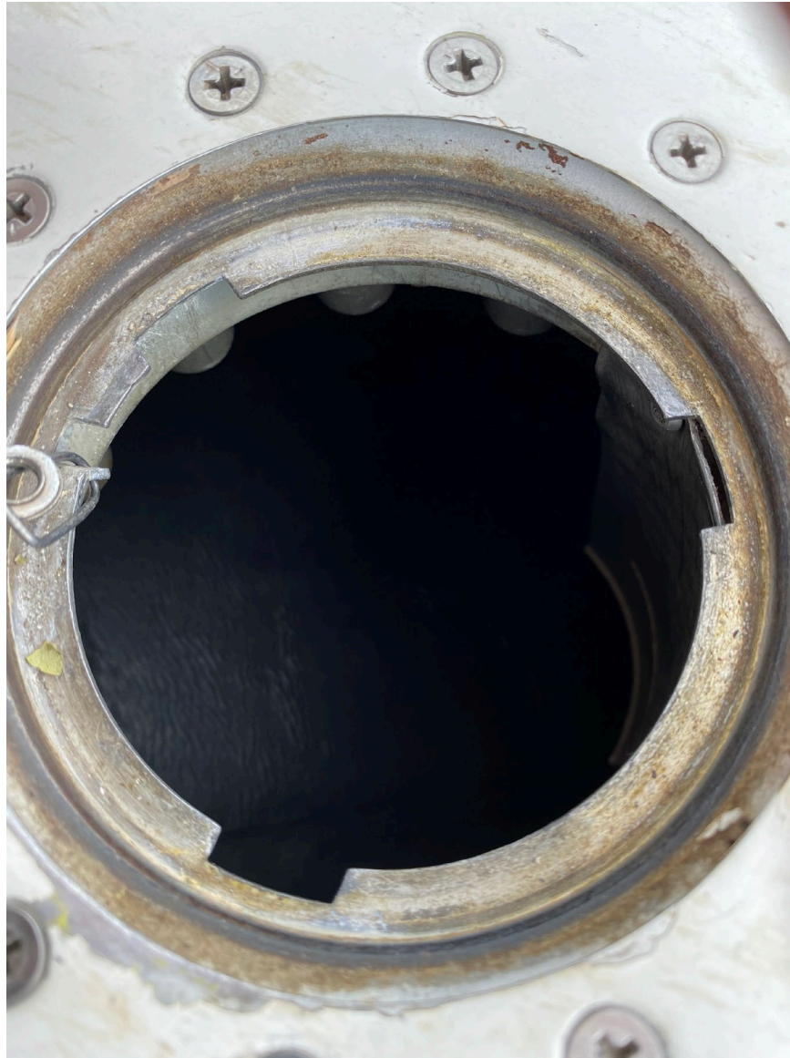
Photograph 2 - Left Wing Fuel Tank Cover (Courtesy of FAA)
