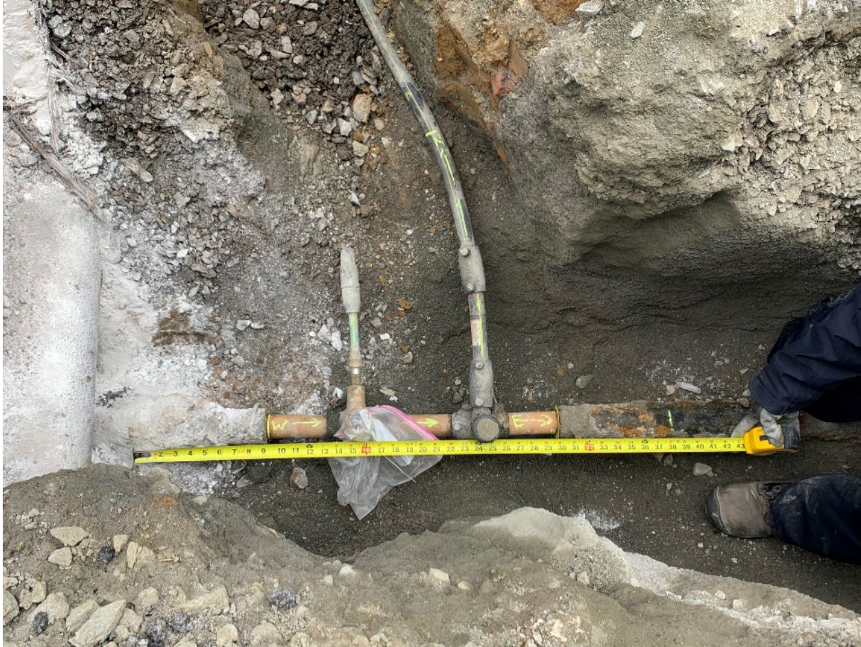
Figure 2. Retired service tee and new service for RM Palmer Building 2
