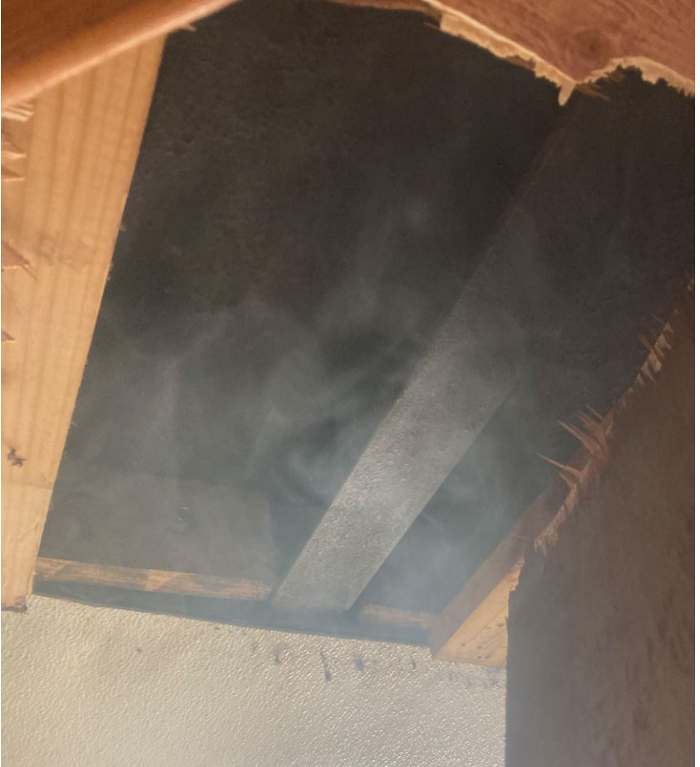
Photo #4 Removed Panel (Ceiling)
