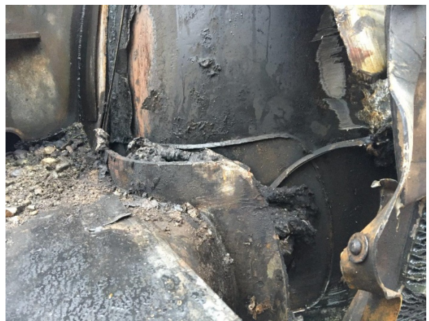
3(f) Separated A-end head pad and fractured fillet weld.
