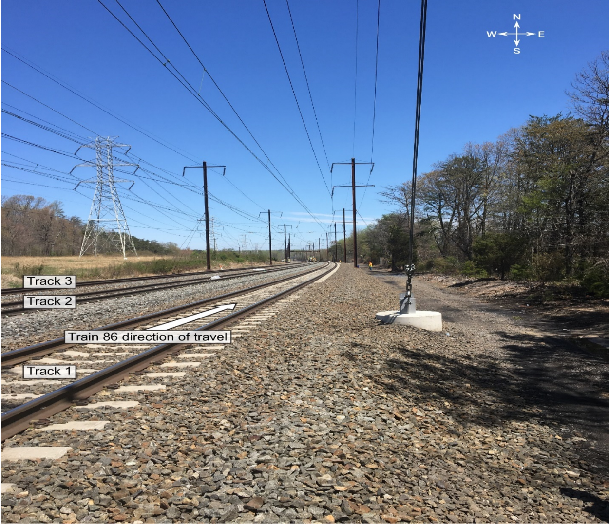
Figure 1- photo taken from Bowie State platform looking north into curve 404. Track 1 is the track to the right of the picture.
