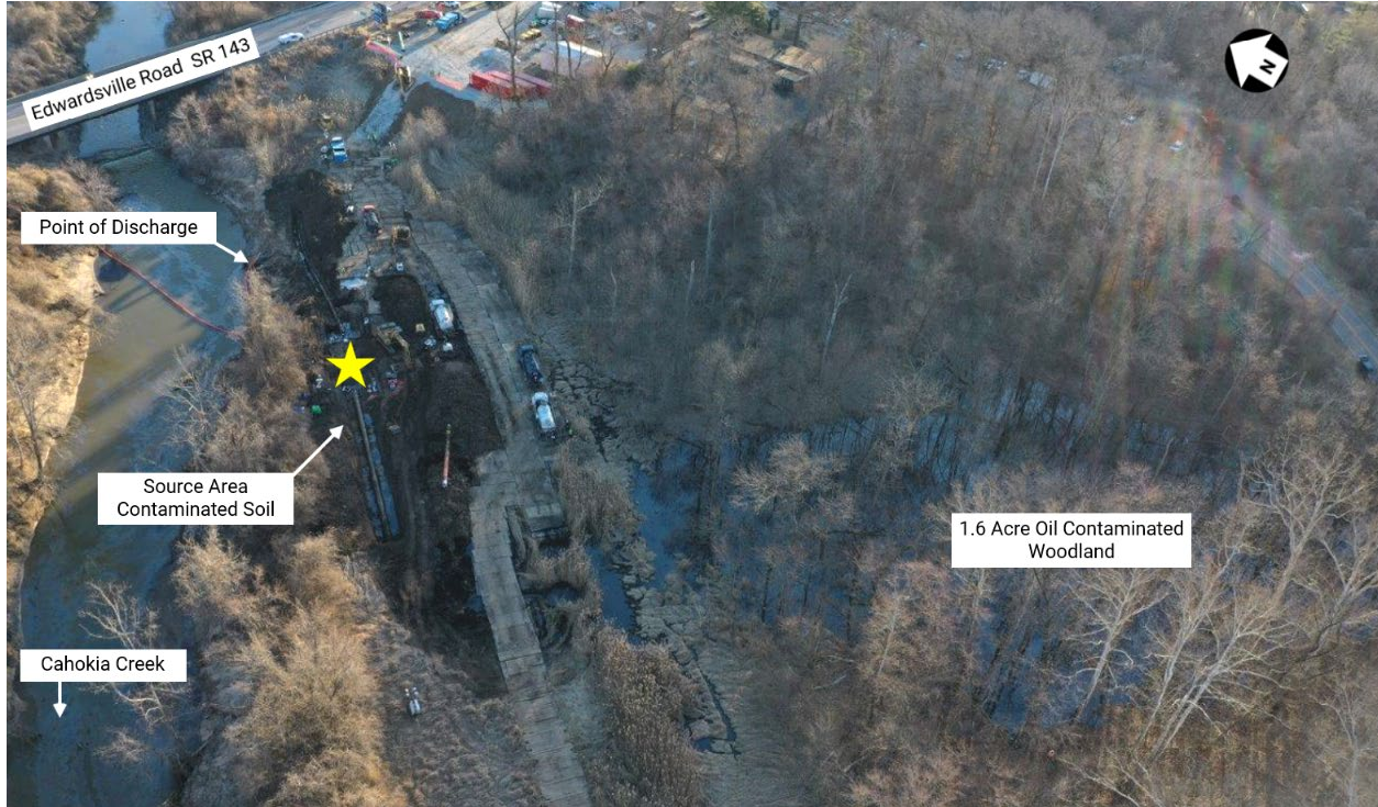
Figure 1. Incident location. Yellow star indicates approximate pipeline breach location. March 13, 2022 at 8:09 a.m. Courtesy of Marathon.
