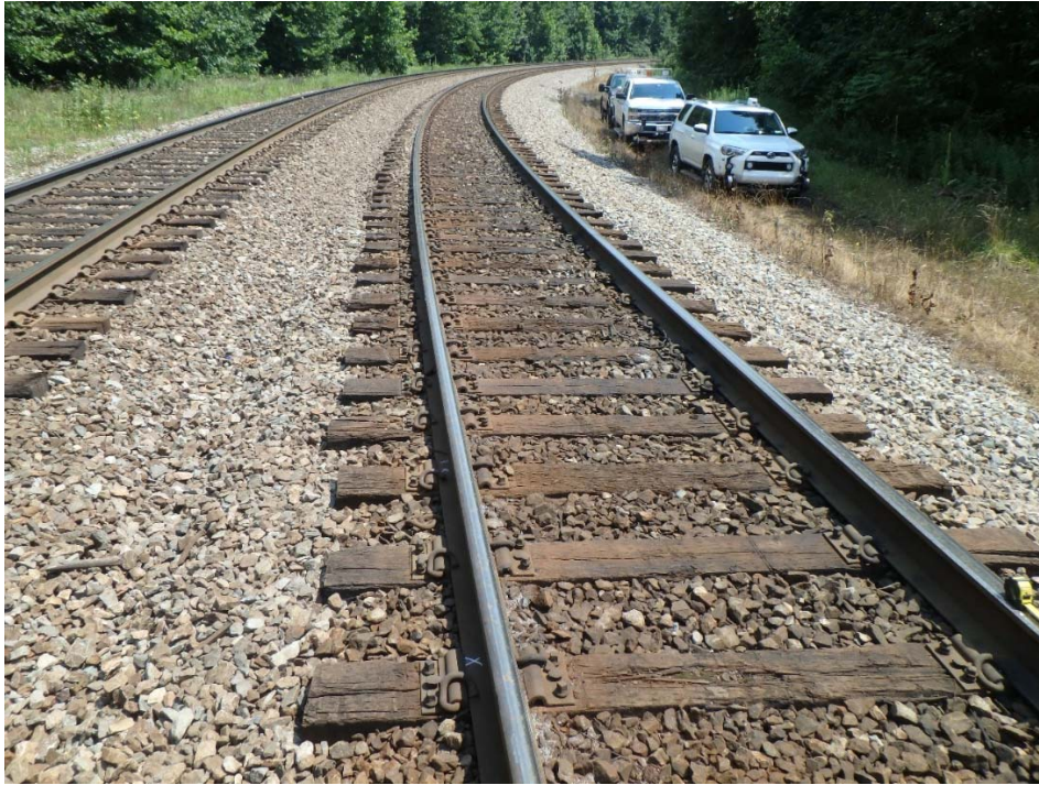
Figure 3. Accident curve facing east toward direction of accident train travel.
