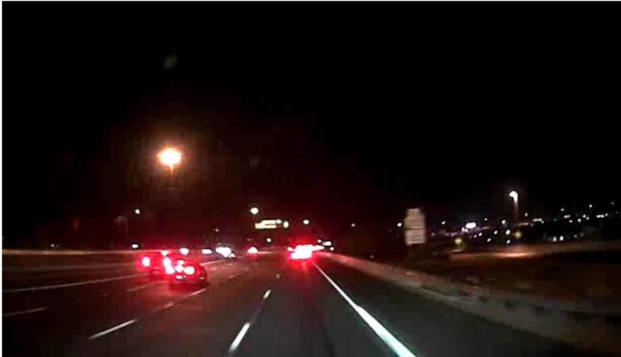
Figure 4. View of highway safety lighting approximately 200-feet west of the impact area. Source: Lytx DriveCam forward-facing in-cab video still image from truck-tractor.
