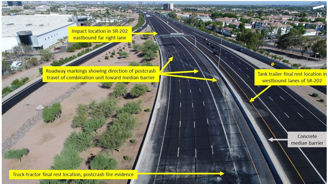
Figure 2. View of the eastbound lanes on the left and westbound lanes on the right in the image with the impact area and tanker positions annotated.
