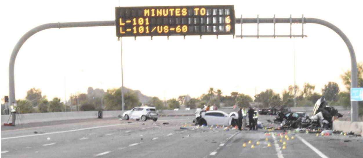
Figure 6. View of permanent DMS board with DTT message at the crash location.
