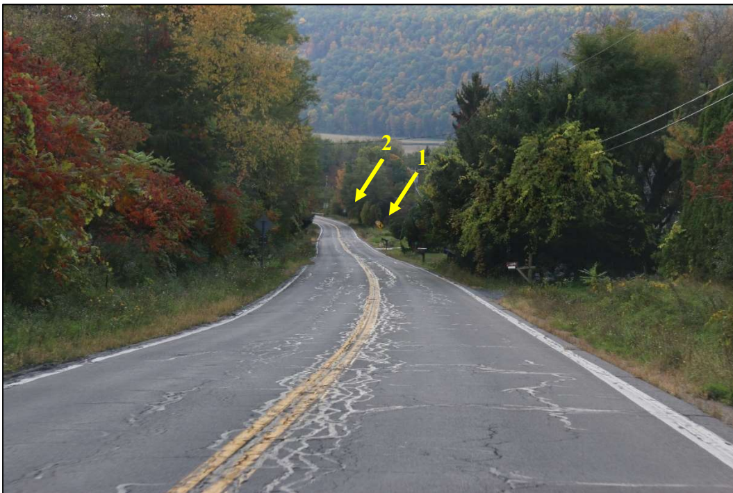
Southbound view of tangent segment following Curve #3 and approaching Curve #4. The signs indicated by yellow arrows include the “Intersection” warning with “Driveways” advisory plaque (#1) and the “Reduced Speed Limit Ahead”, 50-MPH (#2).
