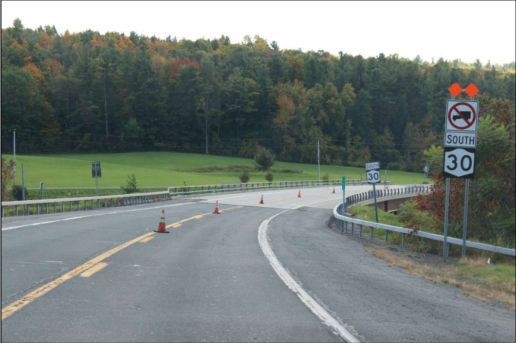
Southbound view along NY-30 through Curve #1 approaching the I-88 overpass. One of the six “No Trucks” is also visible.
