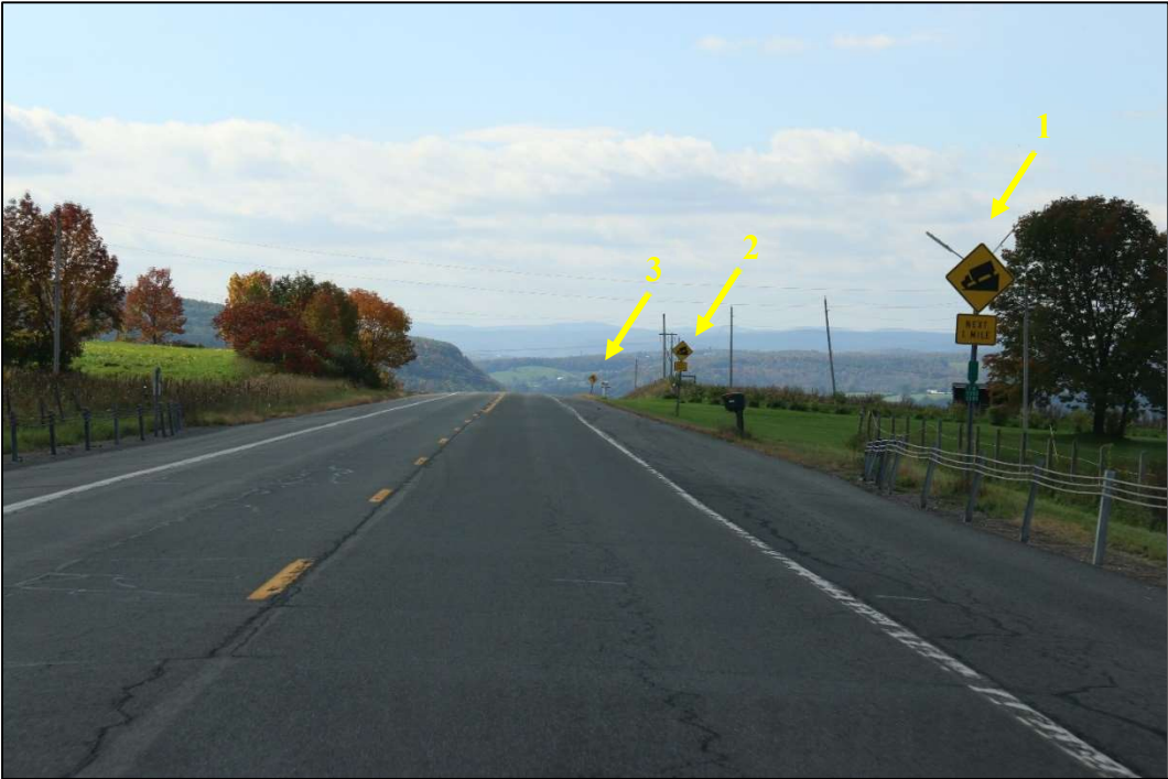
Southbound view after exiting Curve #1 into the tangent segment. The signs indicated by yellow arrows include the first and second “Hill” warning signs (#1 and #2) and the “Curve” warning sign (#3).
