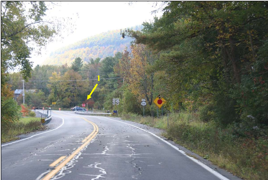
Southbound view approaching Curve #4 and tangent to leading to the NY-30/NY-30A intersection. Visible signs include the “Stop Ahead” sign and intersection “Stop” sign (#1).
