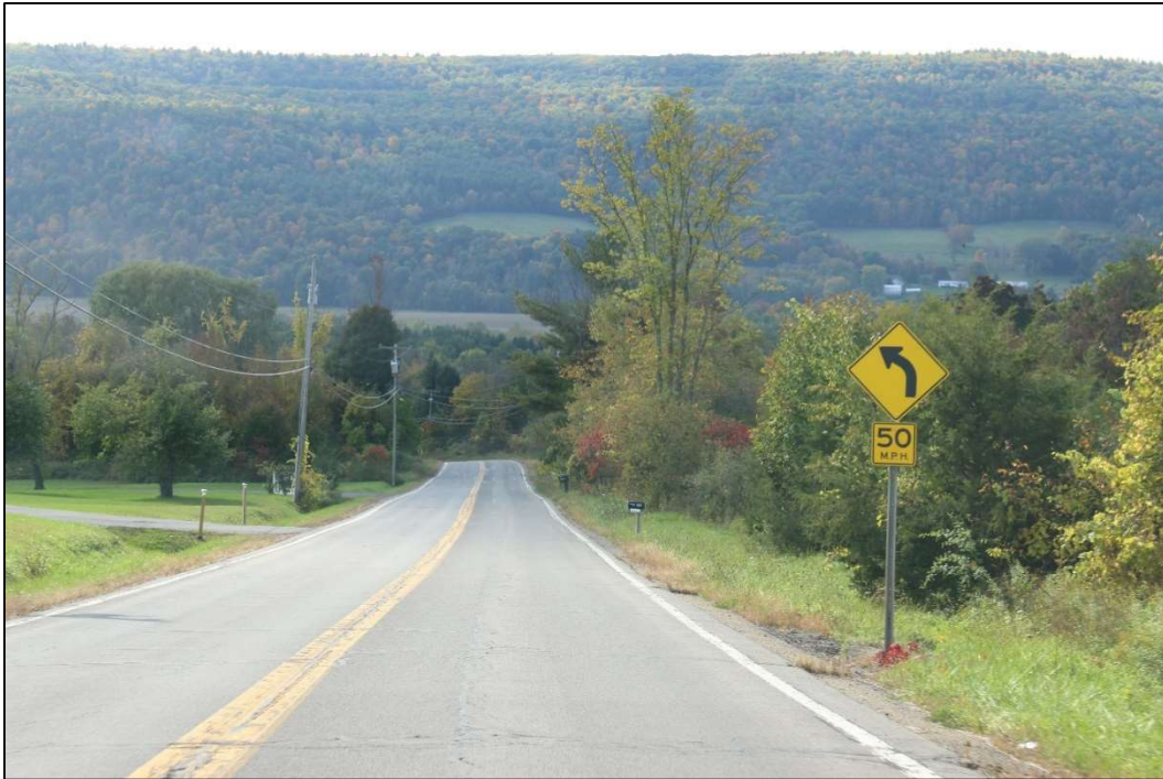
Southbound view along tangent segment approaching curve #3. Image also depicts “Curve” warning sign with reduced speed advisory plaque (50 MPH).
