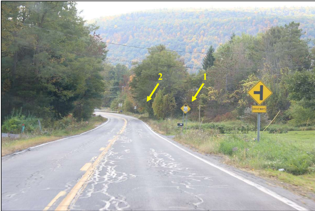
Southbound view approaching Curve #4. Visible signage includes the “Intersection” warning sign, the “Reduced Speed Limit Ahead” sign (#1), and the “Stop Ahead) sign (#2).
