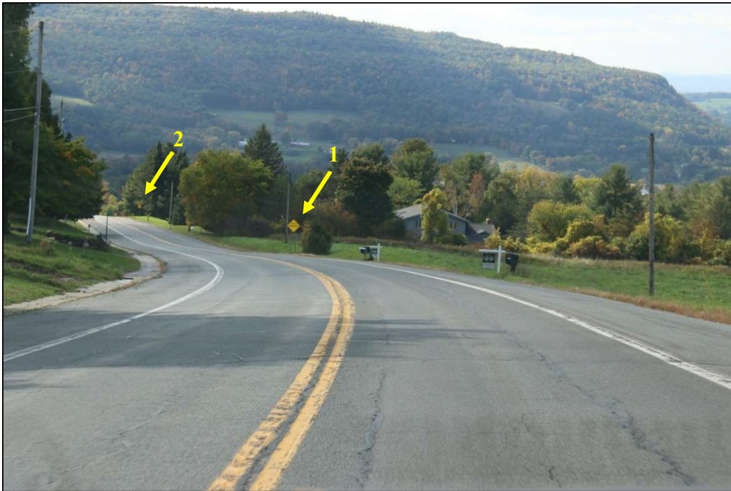
Southbound view toward tangent segment following Curve #2. Signs depicted include "Road Narrows" (#1) and the third "Hill" warning sign (#2).
