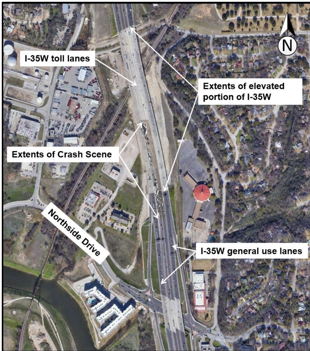
Figure 3 – Extent of the crash scene was approximately 1,100 feet and much of the crash occurred along an elevated 1,900 feet long portion of I-35W (Source: Google Earth image revised).
