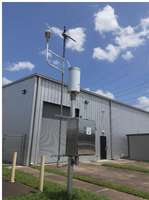
Figure 12 – Environmental Sensor Station (ESS) operated by Houston TranStar (Source: TxDOT).
