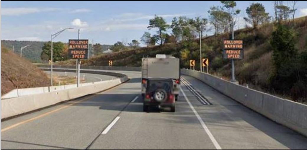
Figure 7 – Automated Truck Rollover Warning System (ATRWS) at the Breezewood eastbound exit ramp.
