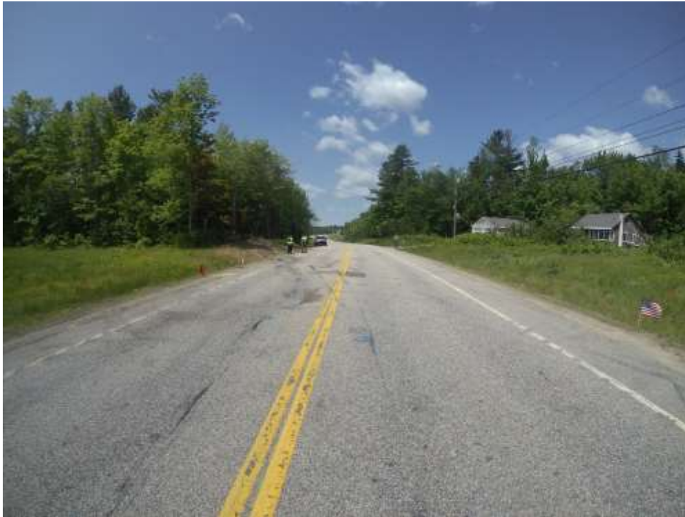
Figure 3 – View of westbound approach to crash location on US Highway 2
