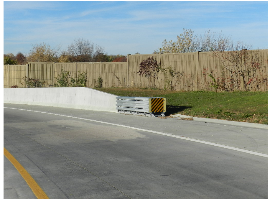
On Ramp to NB US-69
