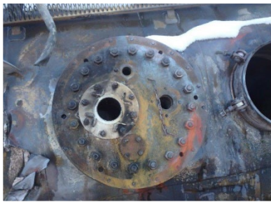
4(a). Top fittings flange, missing protective housing, missing valves and PRD.
