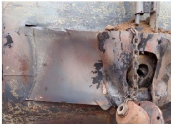
Figure 7. Center skid structure collapse with nozzle assembly sheared as seen hanging by the safety chain. Ball valve partially opened and BOV handle disengaged. CRDX 300056. January 26, 2022. Courtesy Trinity Industries Leasing, Inc.
