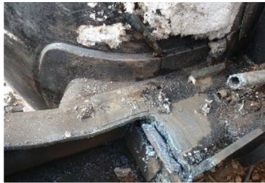
11(d). Repaired B-end right A-2 head pad fillet weld.
