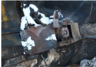
6(b). Buckled tank bottom and BOV skid structure.
