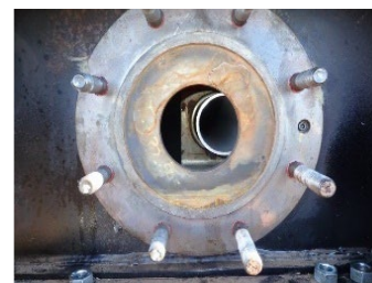
Figure 22. Displaced eduction pipe and flange as seen through BOV hole (Investigators removed the bottom outlet valve from the flange), TILX 731762. January 27, 2022.
