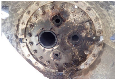
10(a). Top fittings flange after removal of fittings for bench testing.
