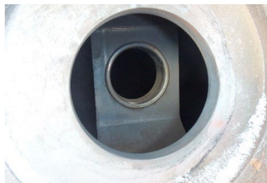
Figure 21. Eduction pipe placement in guide assembly over BOV, TILX 731739. January 27, 2022.
