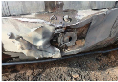
11(a). BOV skid protection structure, shallow dent A-end side (right side in photo).
