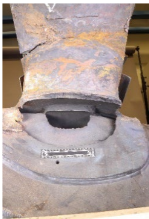
Figure 18. A-end stub sill/head pad/tank section removed for NTSB laboratory examination. TILX 731751. January 28, 2022.
