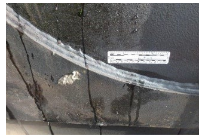
16(f). A-15 inboard sill pad weld.
