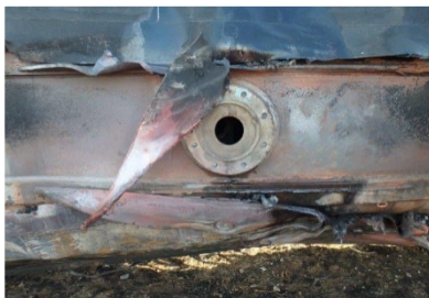
1(a) Missing bottom outlet valve and saddle, and sheared skid protection structure.
