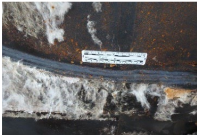
18(a) A-15 weld measurement location.
