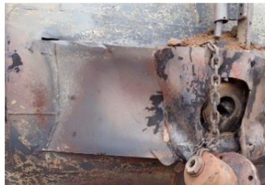
13(b). B-side skid protection structure. Impact marks on right side, dished in the middle. The separated BOV nozzle was hanging from the safety chain.
