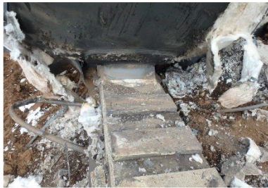
12(b). A-end head pad and head brace, no visible weld cracks.
