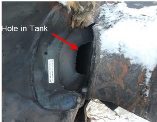
Figure 16. Tank shell breach showing separated head brace and fractured re-pad. TILX731751. January 27, 2022.
